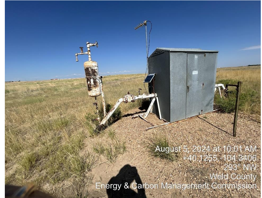
Gas Meter Run & Overgrown Vegetation
