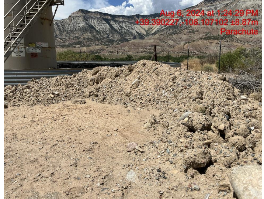
Stockpiled soils with no BMP's - Photo #04277
