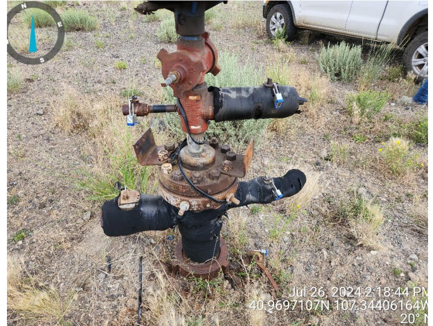
Five ECMC locks installed on valve handles.
