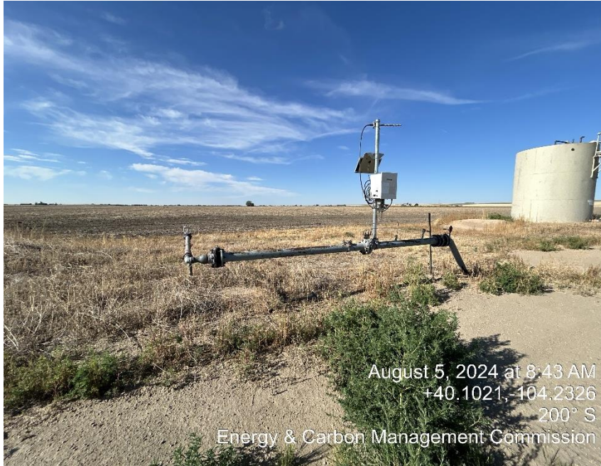
Sirius Brothers Gas Meter Run
