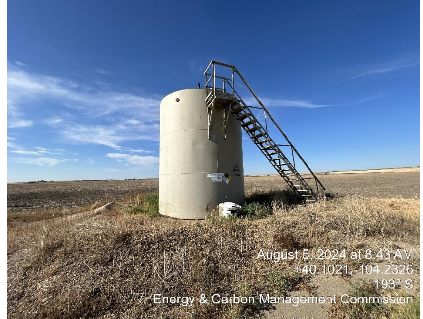
Crude oil tank
