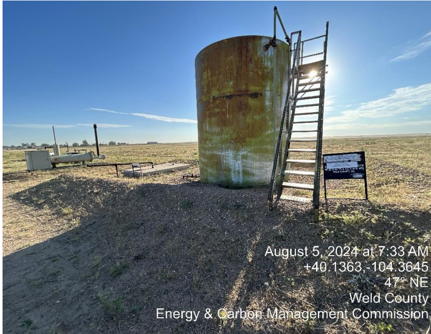
Crude tank & needs NFPA Placard & capacity label
