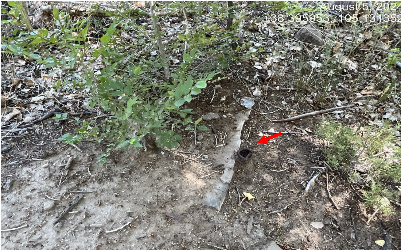
Photo 3. Facing southwest at the abandoned wellsite. There is a pipe at red arrow and wood block. Previous corrective action was not completed.
