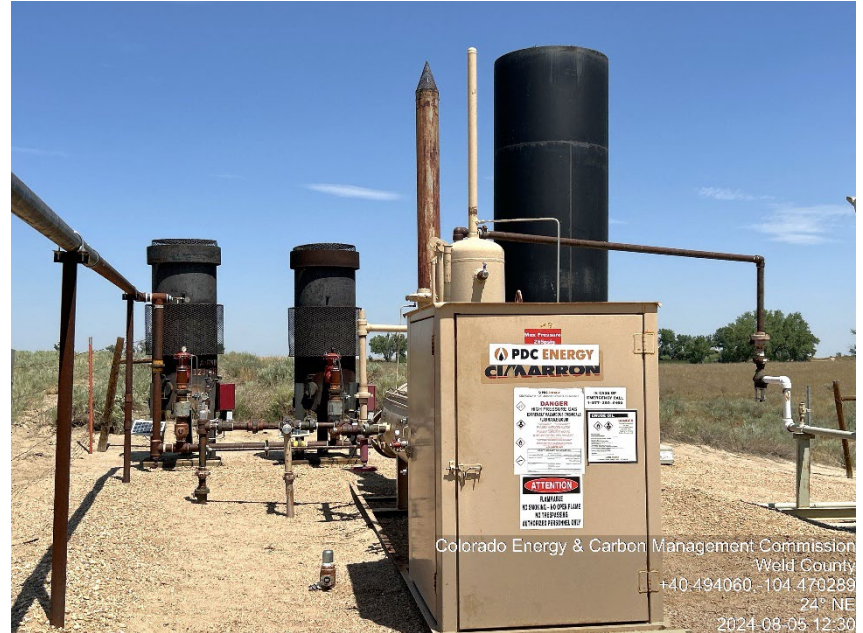
Photo #4 Cornish 14-8 Battery site Active ECD(s), Separator(s)
