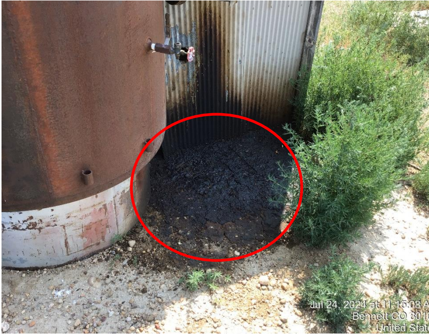
Photo #3 Stained soil on back side of the separator.
