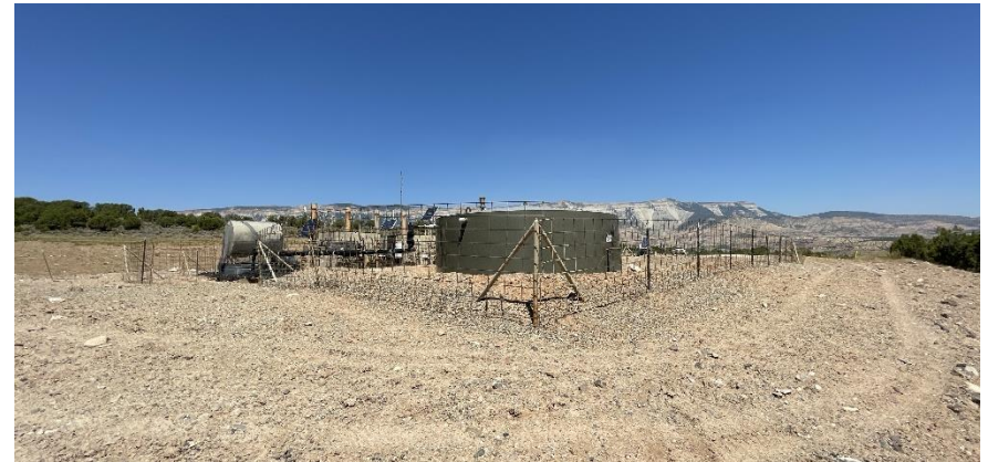
South East corner of location.
