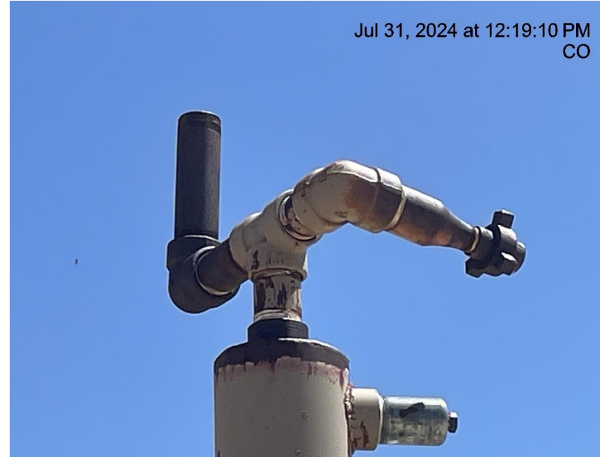
Photo # 4251 Open ended piping/wildlife hazard
