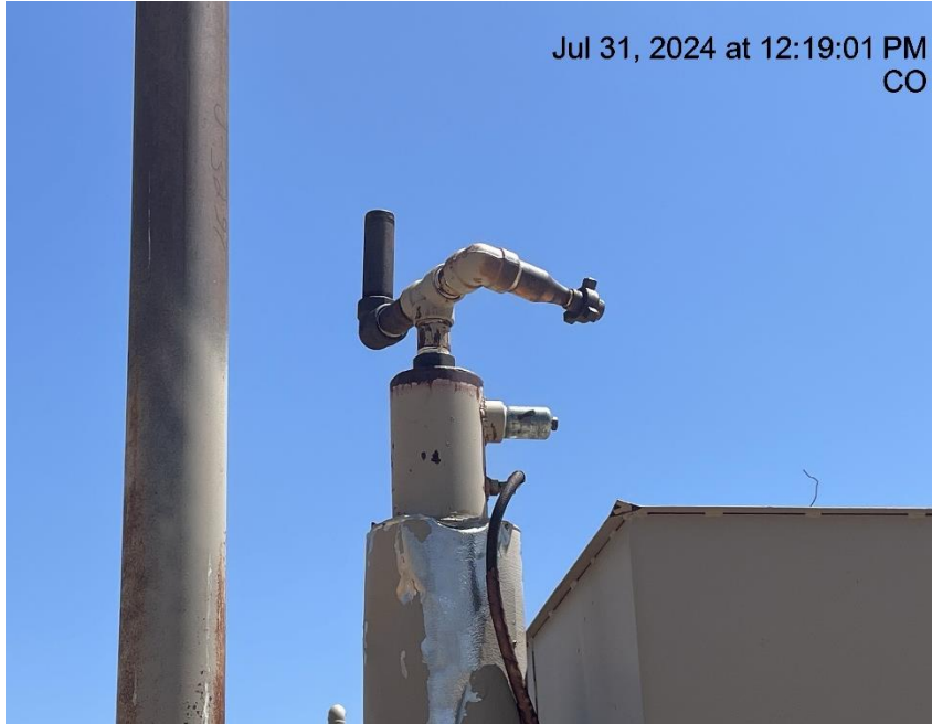
Photo # 4250 Open ended piping/wildlife hazard
