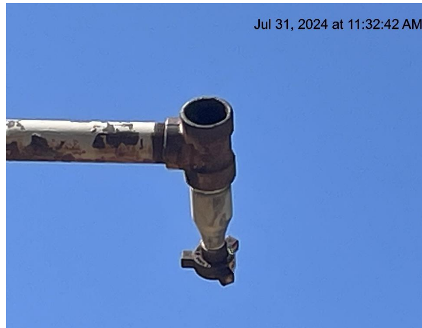
Photo # 4204 Open ended piping on separator unit/wildlife hazard
