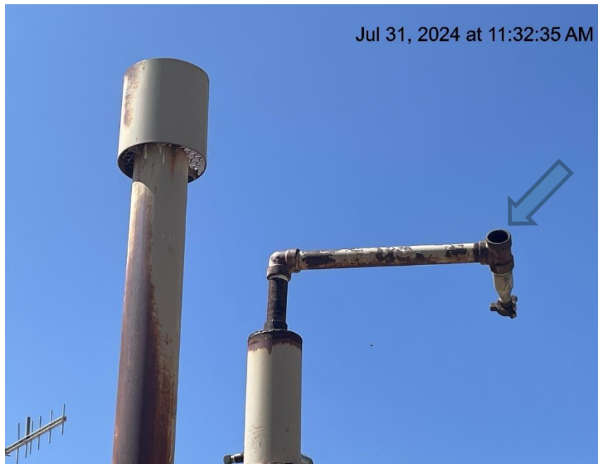
Photo # 4203 Open ended piping on separator unit/wildlife hazard
