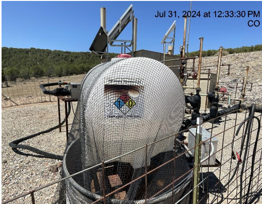
Photo # 4283 Chemical tank label weathered & some required info is illegible/does not comply with CECMC rules
