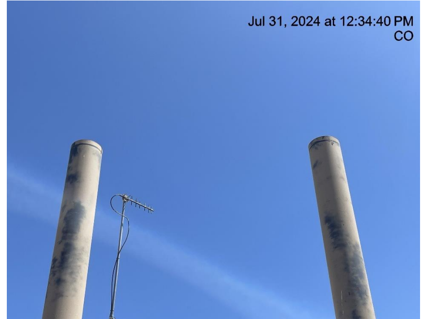
Photo # 4282 Burner exhaust stacks on separator unit lack bird protection
