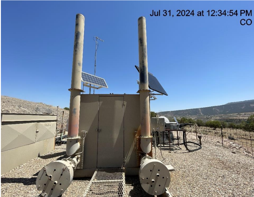
Photo # 4281 Burner exhaust stacks on separator unit lack bird protection
