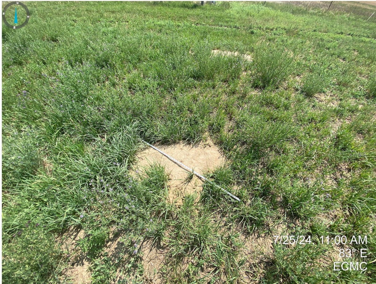
Photo 2. Subsidence around flowline potholes appears to have been backfilled and leveled.
