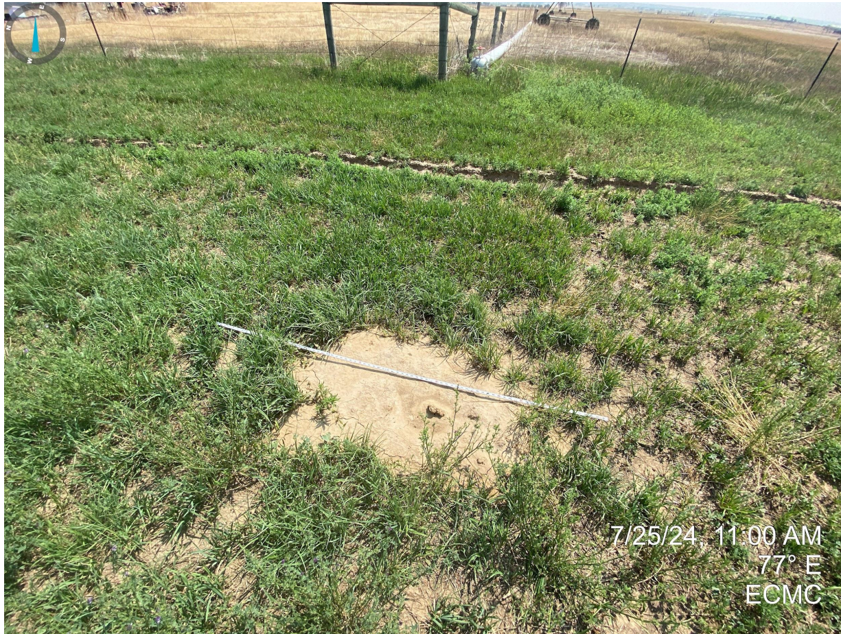
Photo 3. Subsidence around flowline potholes appears to have been backfilled and leveled.
