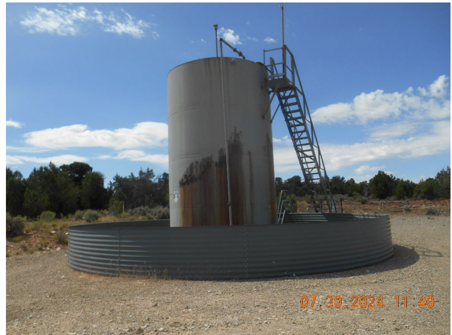
Tank Battery Rusted out
