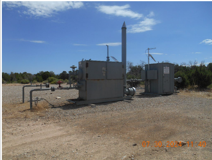
Separator and Meter housing
