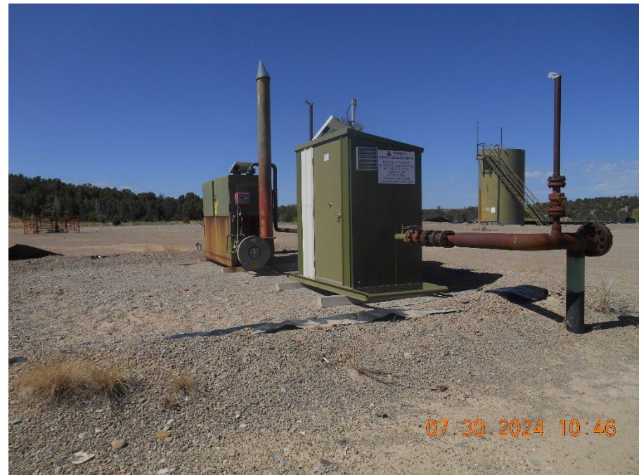
Separator and Meter housing
