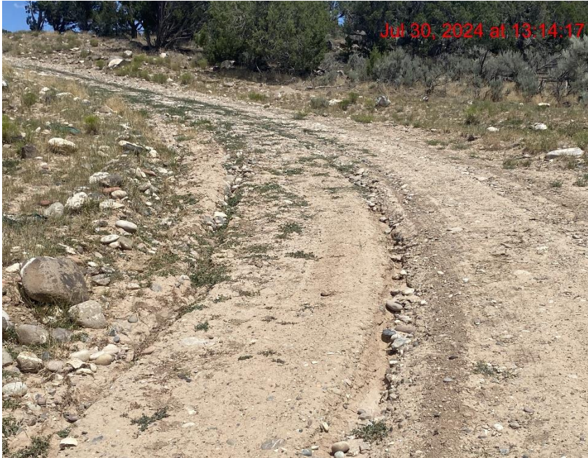
Insufficient Erosion Control/Rill Erosion – Photo #02493
