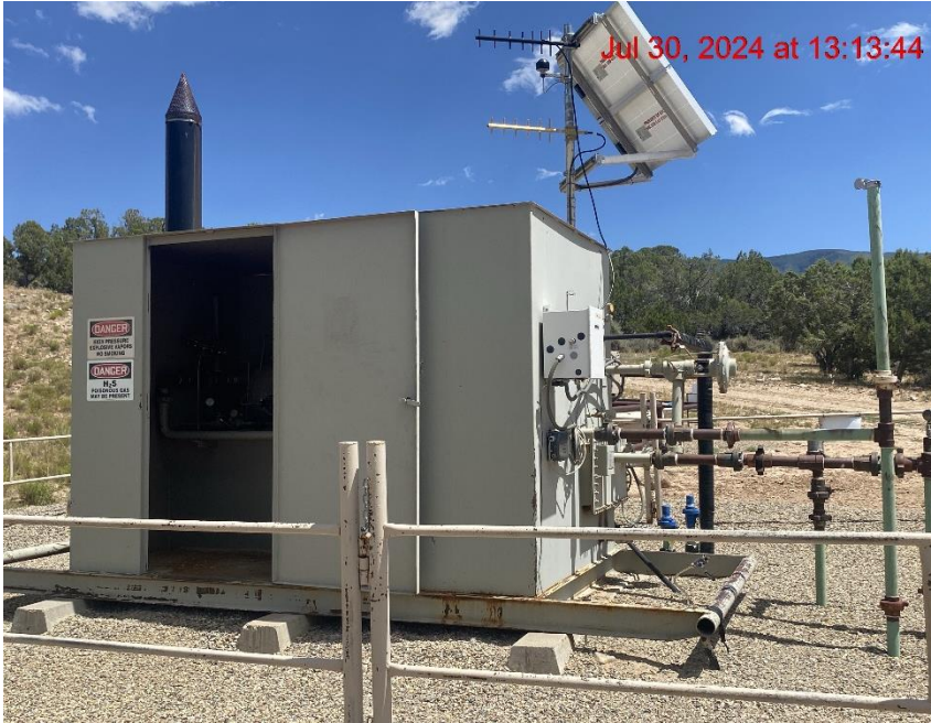
Unsecured Separator – Photo #02492
