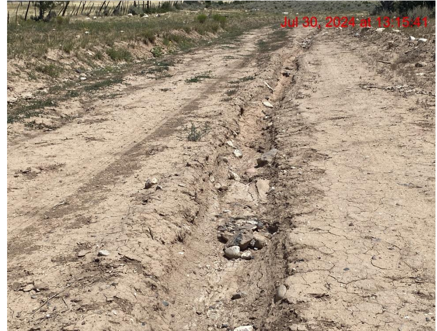
Insufficient Erosion Control/Rill Erosion – Photo #02494
