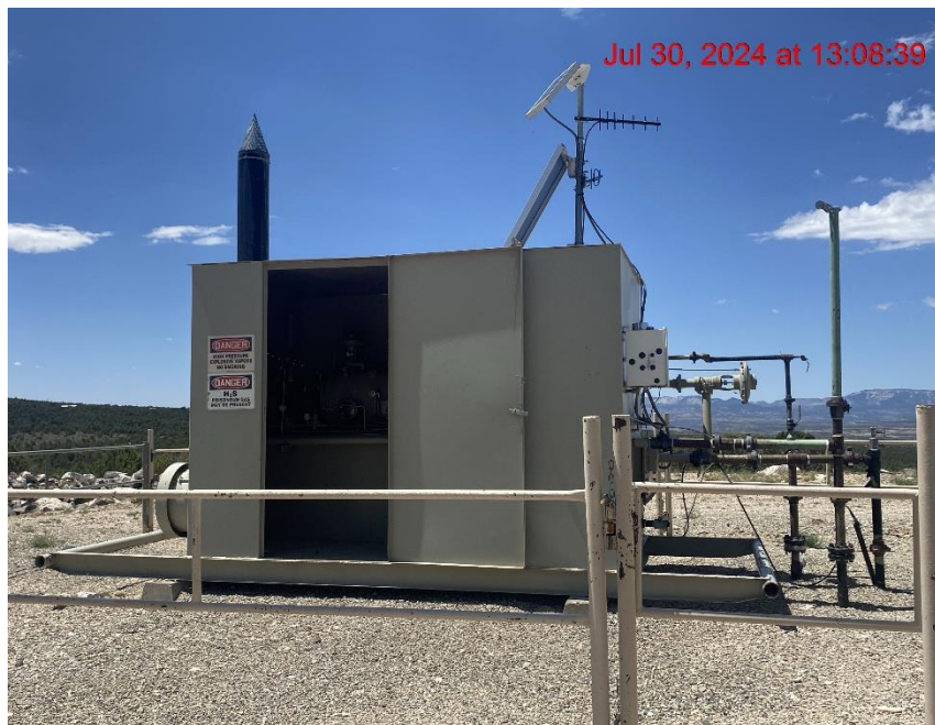
Unsecured Separator – Photo #02485
