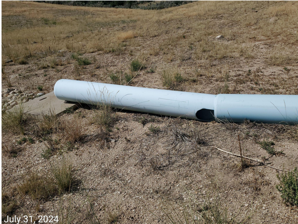
Photo 8: Photo shows slope drain in disrepair.
