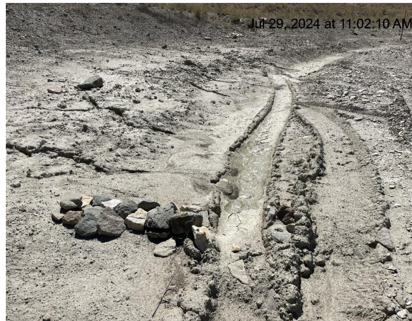
Photo # 3782 Vehicle tracks observed in ditch & some damage observed to check dams in ditch
