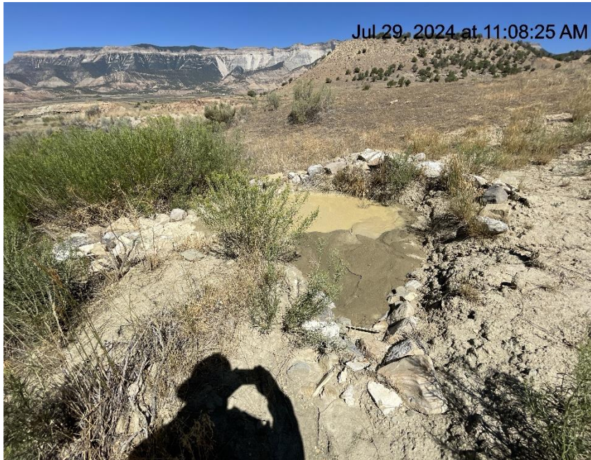
Photo # 3785 Sediment trap approximately 90% full & may need maintenance in near future (N/NW area of location)
