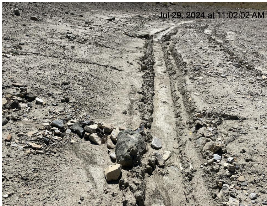
Photo # 3781 Vehicle tracks observed in ditch & some damage observed to check dams in ditch
