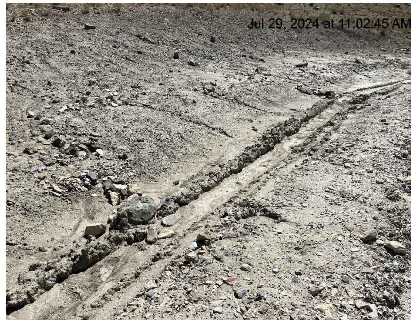
Photo # 3784 Vehicle tracks observed in ditch & some damage observed to check dams in ditch
