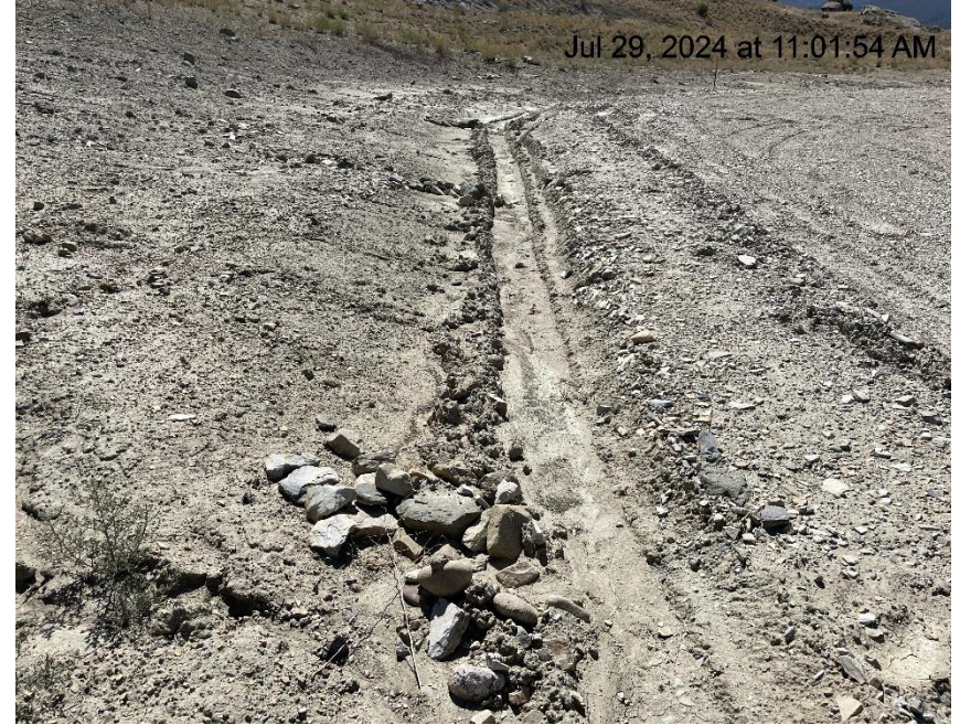
Photo # 3780 Vehicle tracks observed in ditch & some damage observed to check dams in ditch
