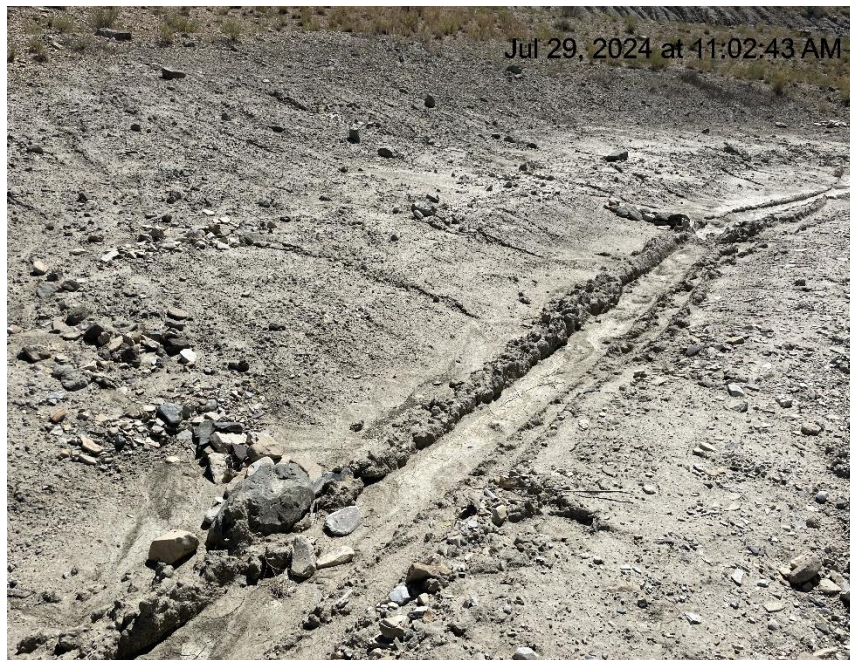
Photo # 3783 Vehicle tracks observed in ditch & some damage observed to check dams in ditch
