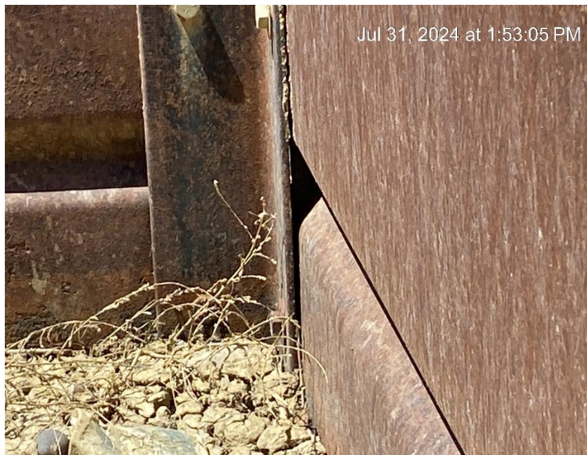
Unsealed tank berm
