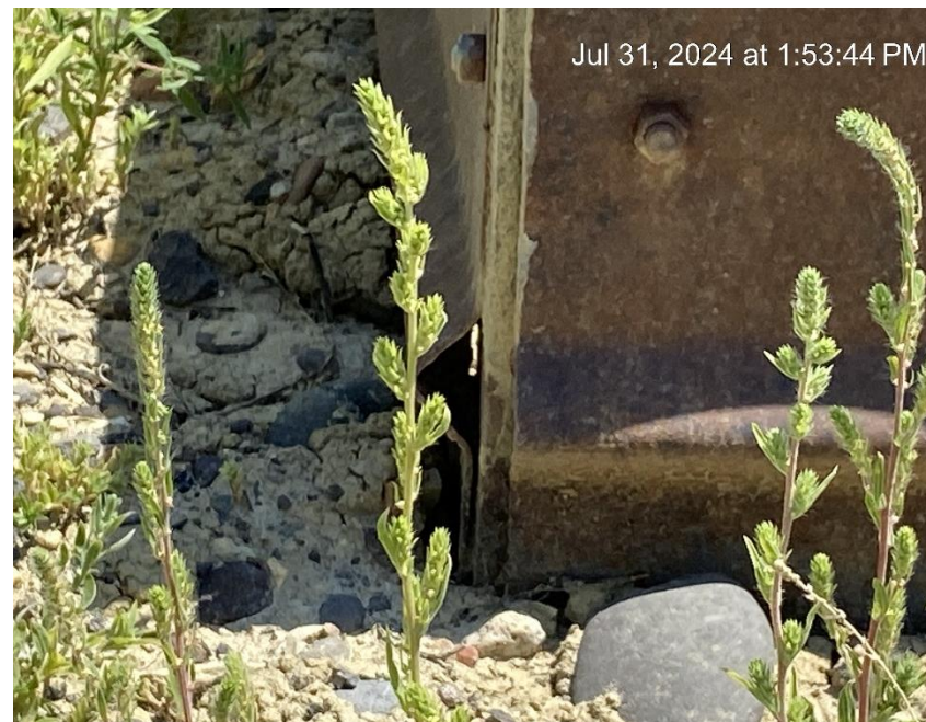
Unsealed tank berm
