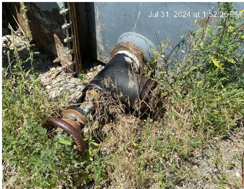
Leak and stained soil
