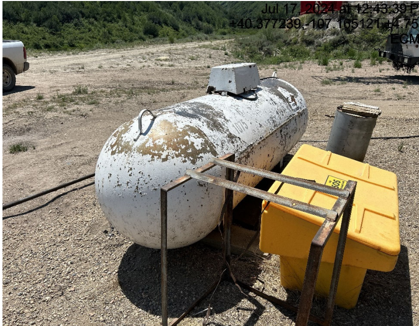
Tank missing proper labeling
