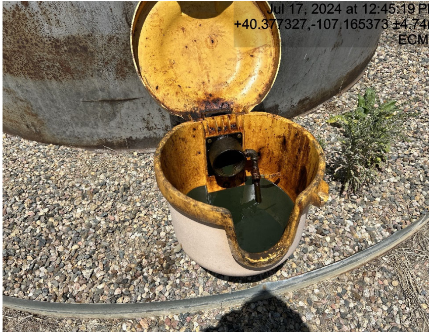
Load line missing cap/plug
