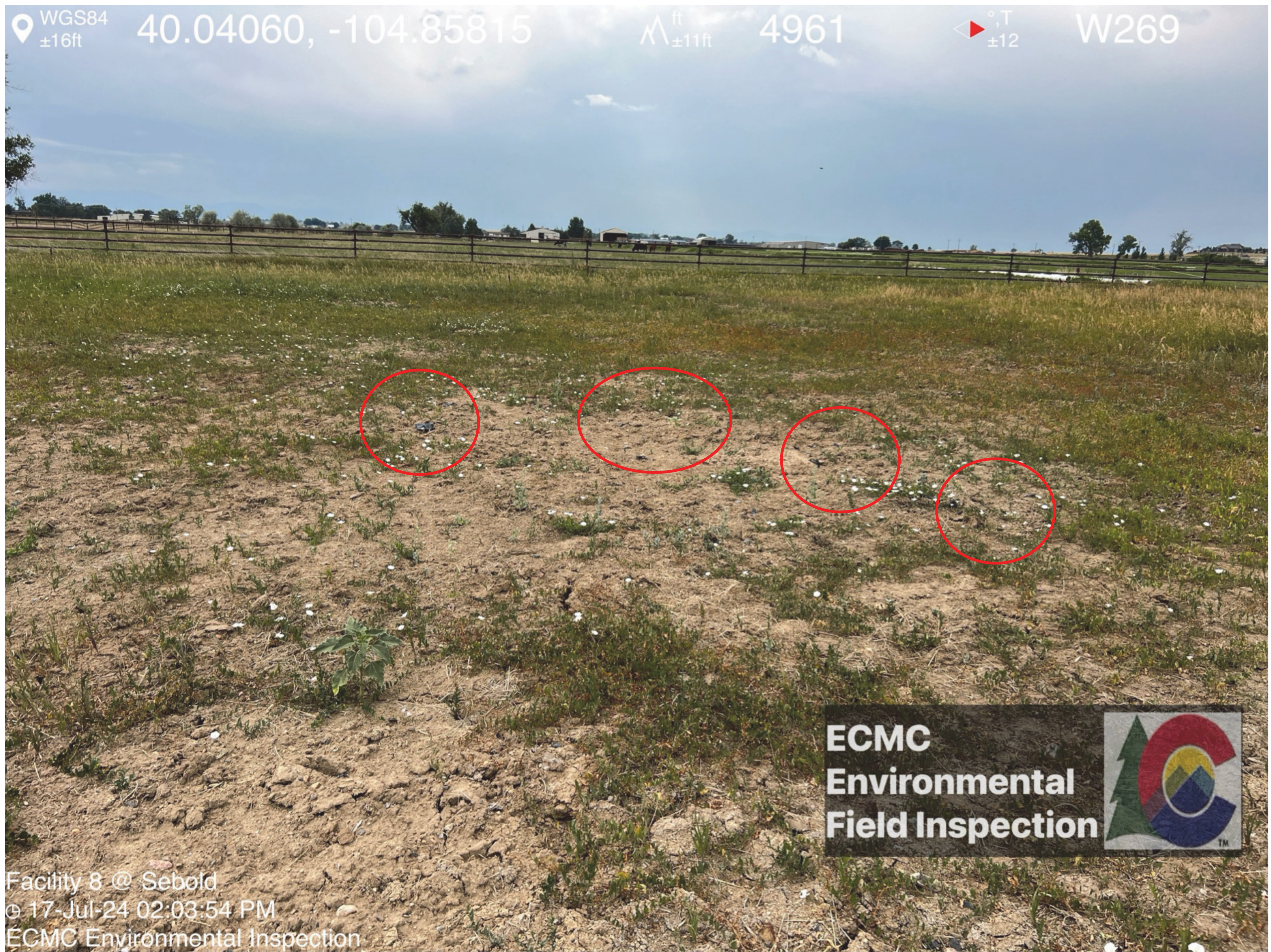
Weeds/Debris/Trash. Footprint of work area/former stockpile. Pieces of former E&P Waste Stockpile liner and trash observed throughout work area.
