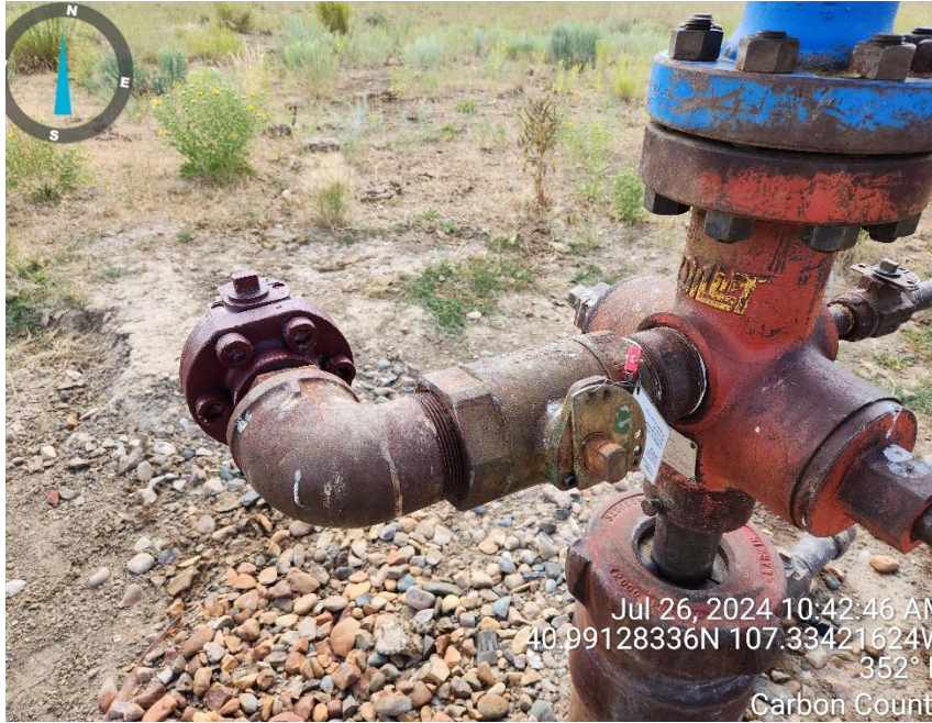
BLM tag remains on 2" valve upstream of recently installed 2" valve and plug.
