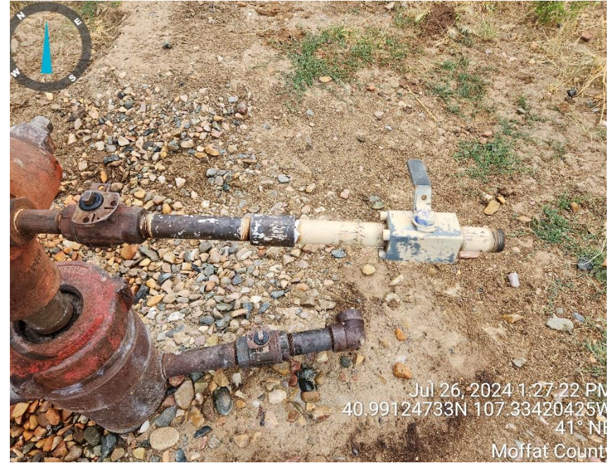
During this inspection, ECMC staff installed a 1" valve to stop leak.
