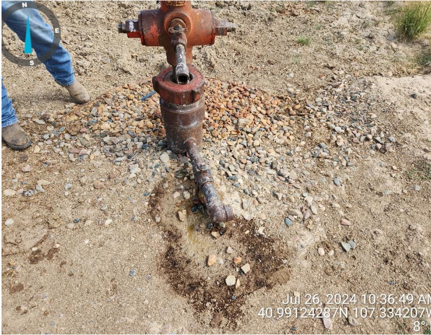
The 1" valve was leaking during this inspection.
