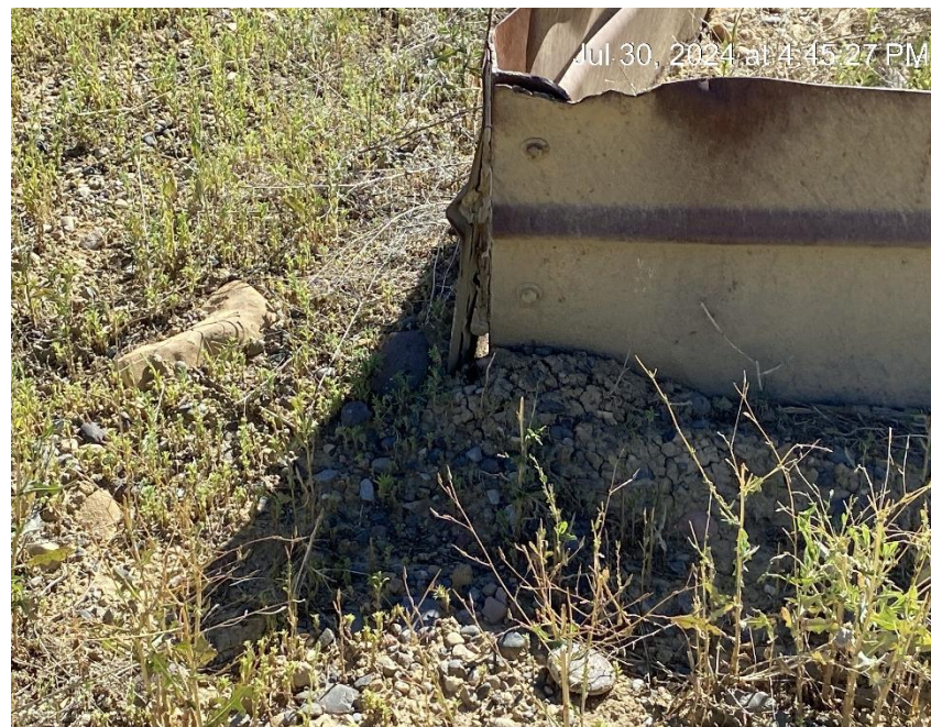
Damaged tank containment with hole
