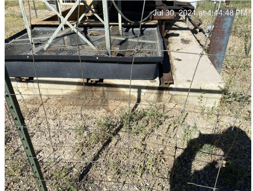
Equipment leakage and stained soil
