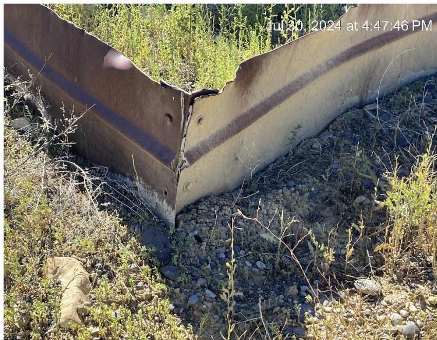
Damaged tank containment
