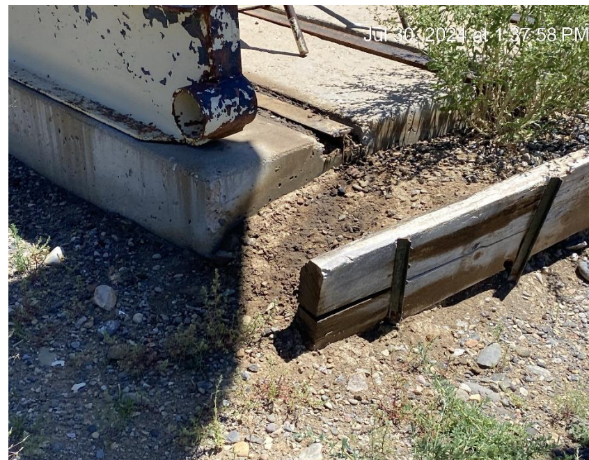
Leaking equipment and stained soil
