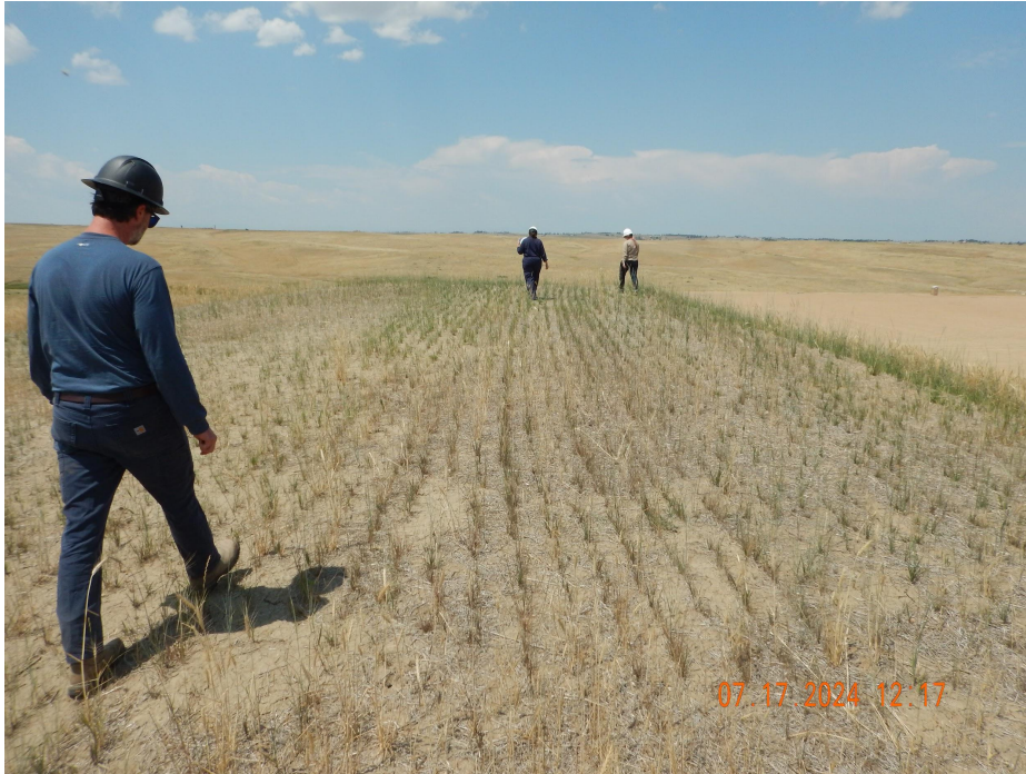
Photo 8. Photo taken from the southern perimeter, facing West. Photo illustrates the southern perimeter which is has a cut slope on the eastern half and fill slope on the western half.
