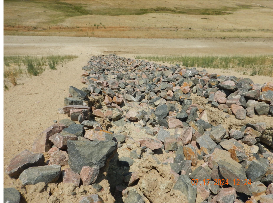
Photo 11. Photo taken from the western working pad surface, facing West. Photo illustrates a stabilized channel that is directed to a retention pond. The riprap was not lined underneath; therefore, stormwater erosion is undermining the riprap. CDPHE will be addressing this corrective action.
