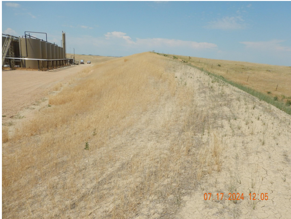
Photo 6. Photo taken from the northeastern perimeter, facing West. Photo illustrates the northern perimeter which is mostly a cut slope that is in process of being stabilized with vegetation.
