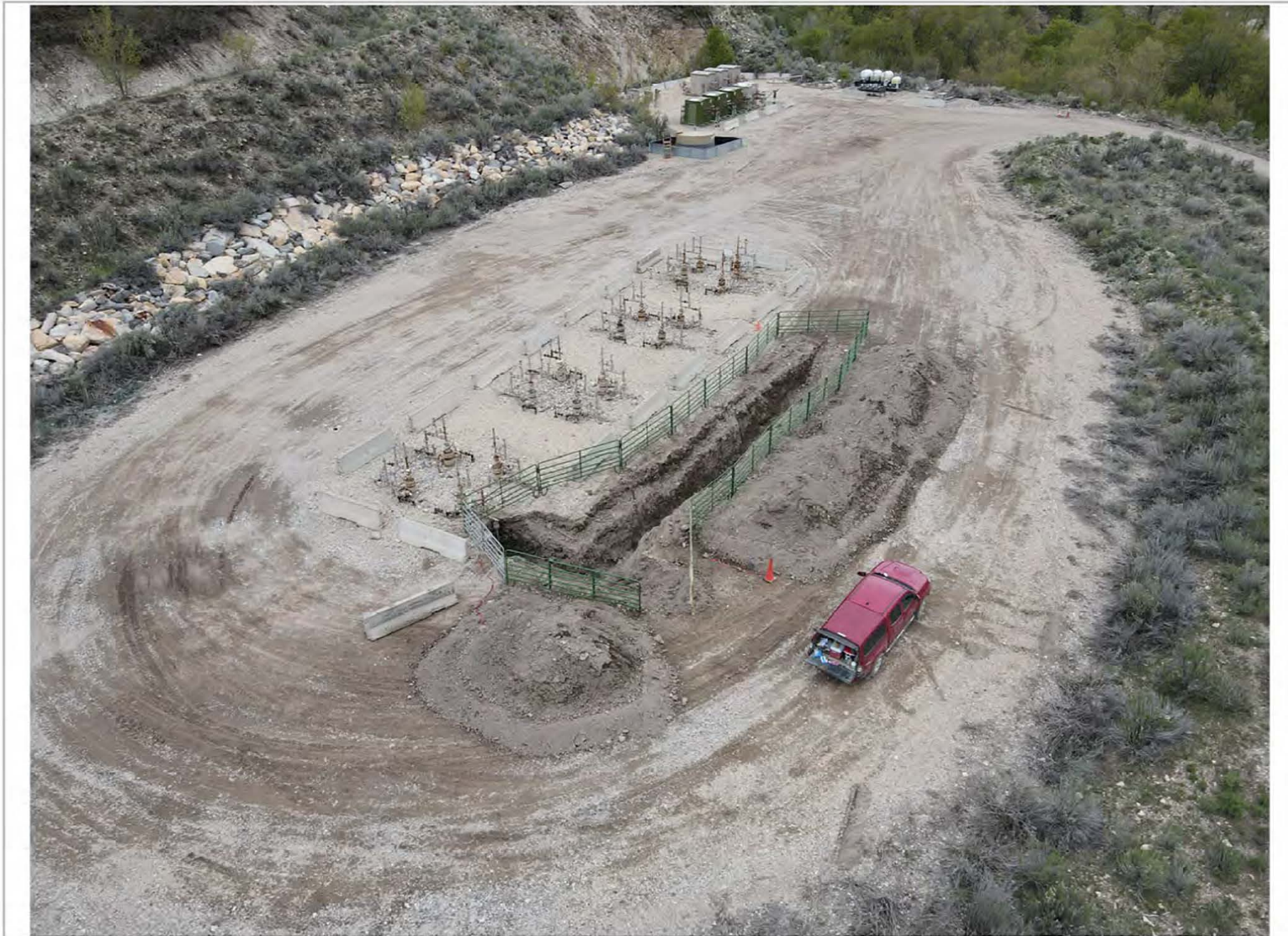
L29 595 Excavation: View Southwest
