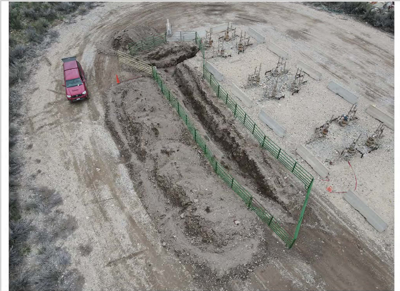
L29 595 Excavation: View East
