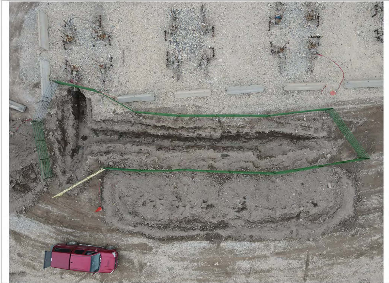
L29 595 Excavation: Orientation Southeast
