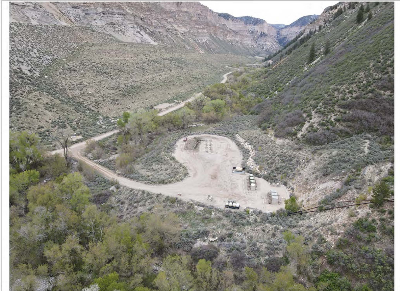
L29 595 View: Northeast
