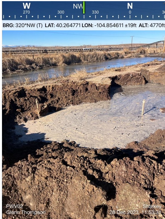
PWV 02 Excavation (Groundwater Present in Excavation)
