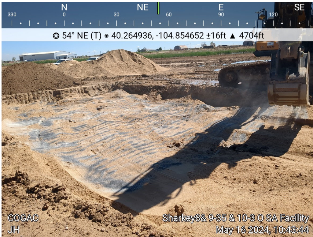
Backfill in process
