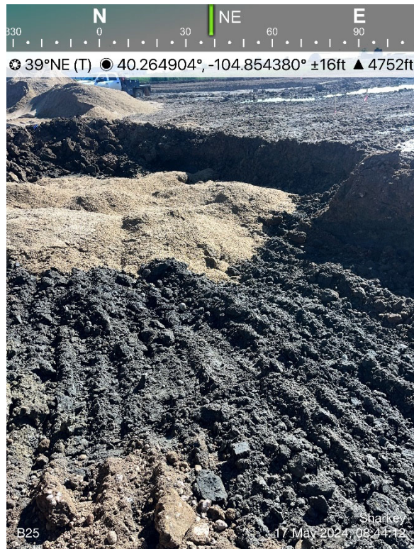
B25 Backfill in process
