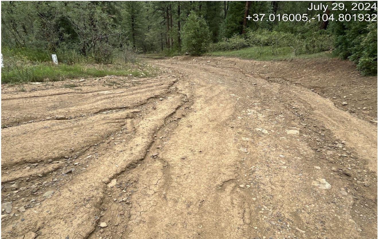
Photo 3. Facing back down the road at the wellsite. There is erosion occurring down the road causing erosion. A berm would help divert the water off the road to prevent erosion.
