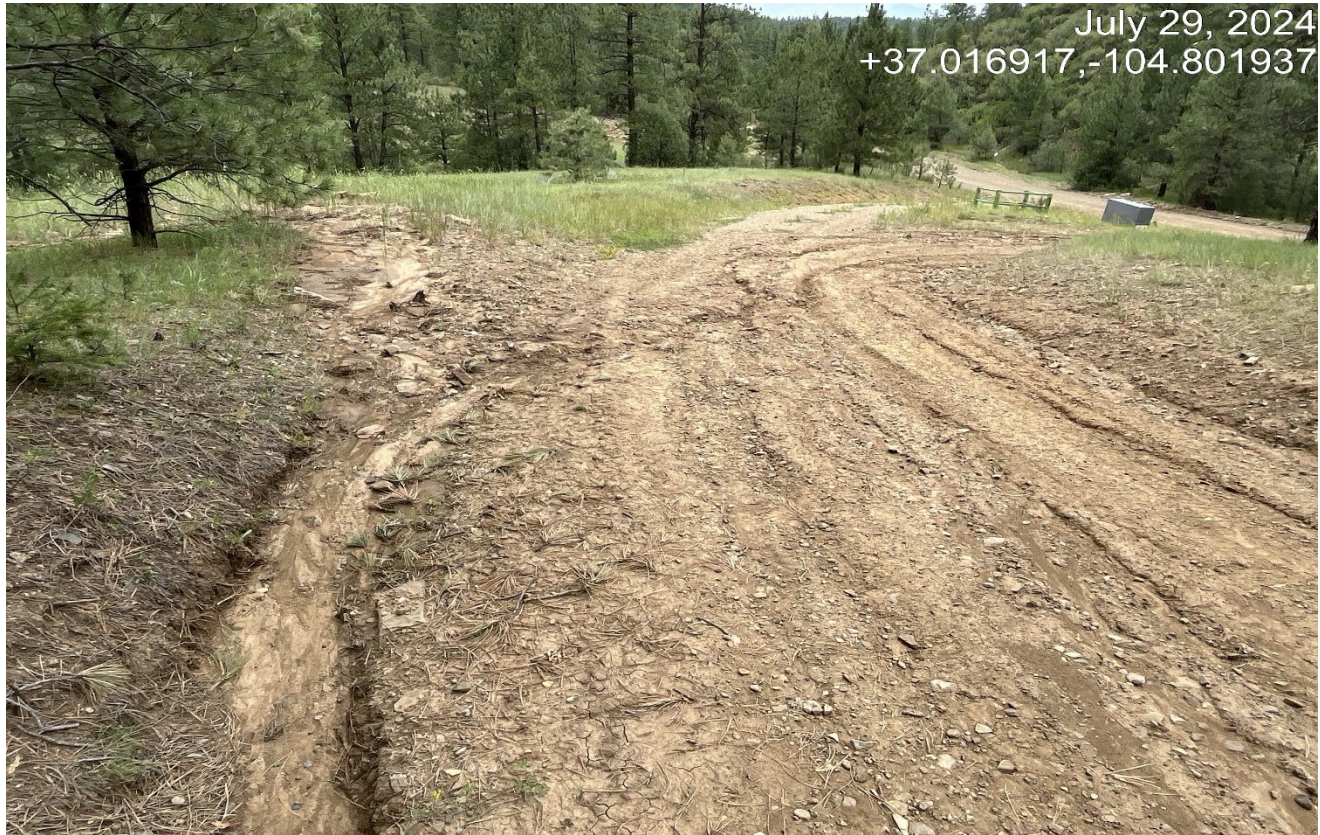
Photo 2. Facing northeast along the access road. Sediment has filled into the diversion ditch and stormwater is going back onto the road causing erosion..
