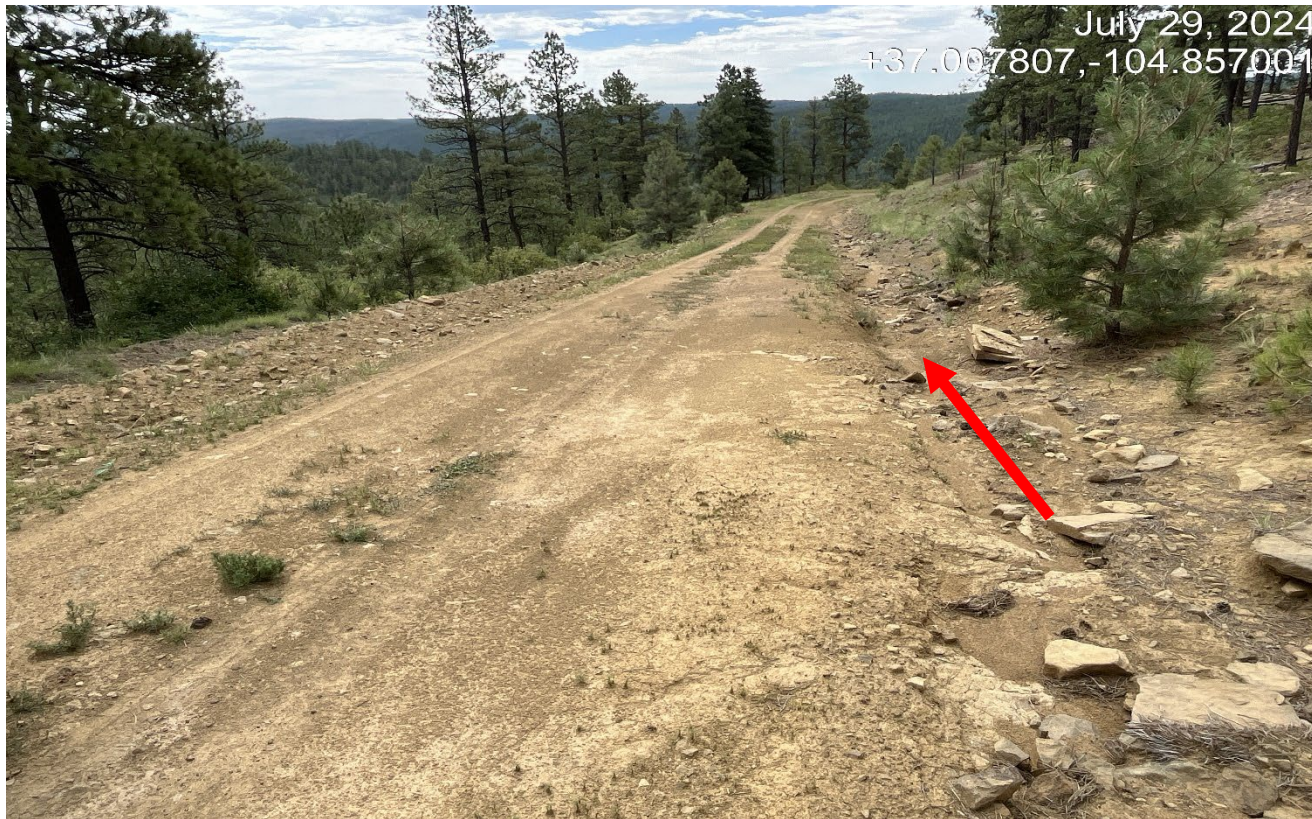
Photo 1. Facing northeast along the access road. There is a long stretch of road with no stormwater diversion which is concentrating a lot of flow to the area in the following pictures.
