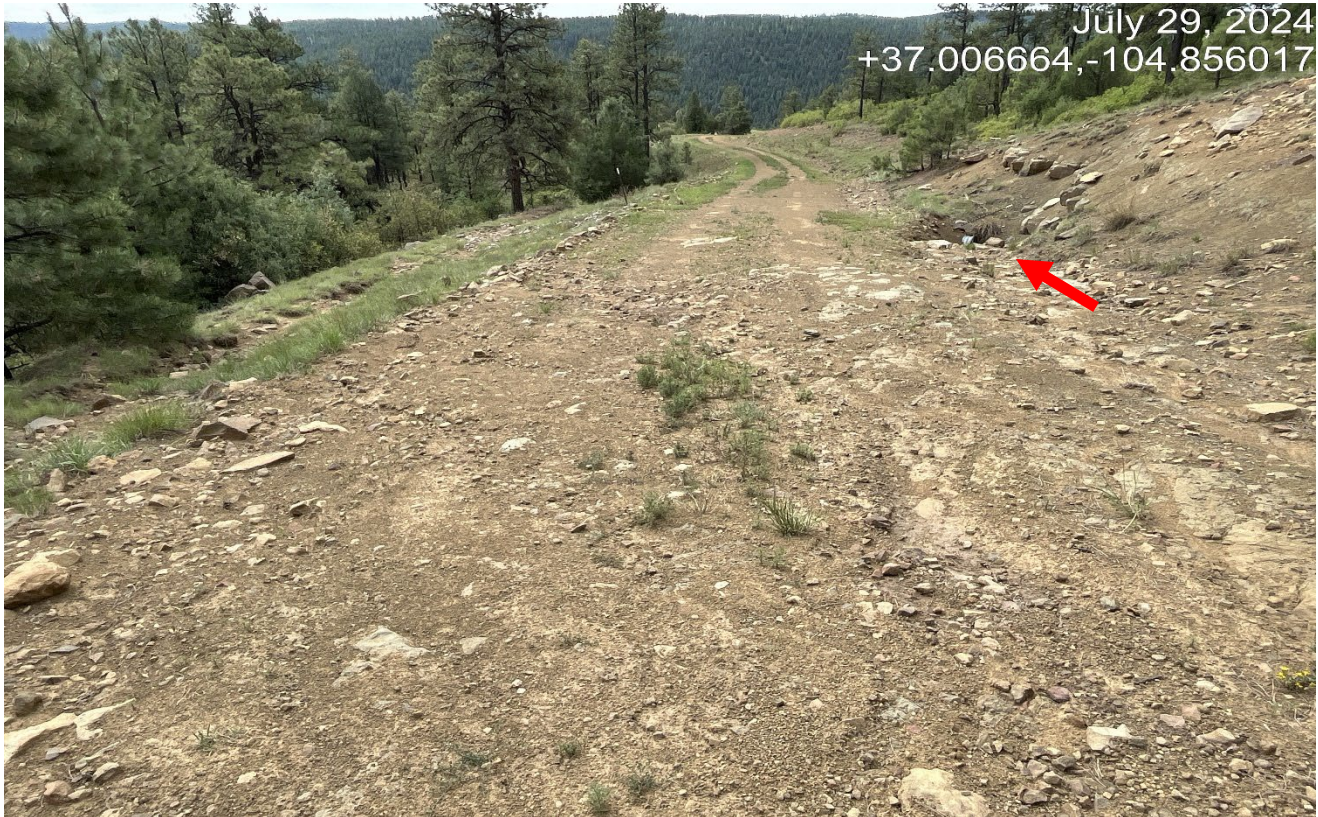
Photo 3. Stormwater is flowing across the road instead of toward the culvert at red arrow.
