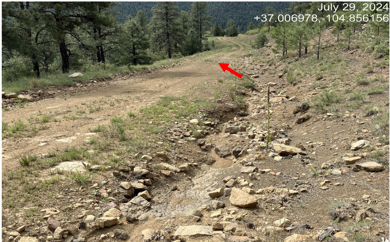
Photo 2. Facing southeast along the access road. There is erosion along the roadside which needs BMP's to control erosion. Tip: Rocks could be utilized to create check dam structures for erosion control.
