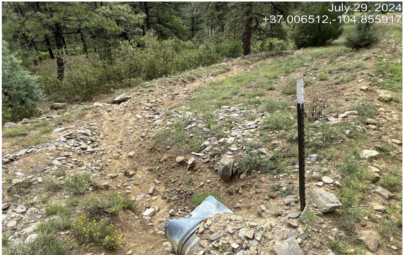
Photo 4. The culvert does not have outlet protection and erosion is occurring in this area.
