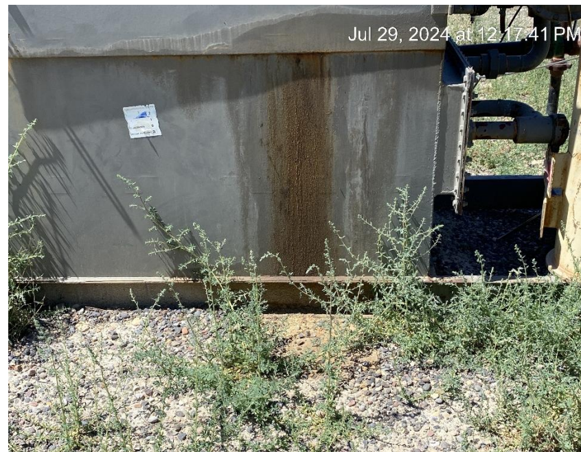
Leaking equipment. Oily waste and staining.
