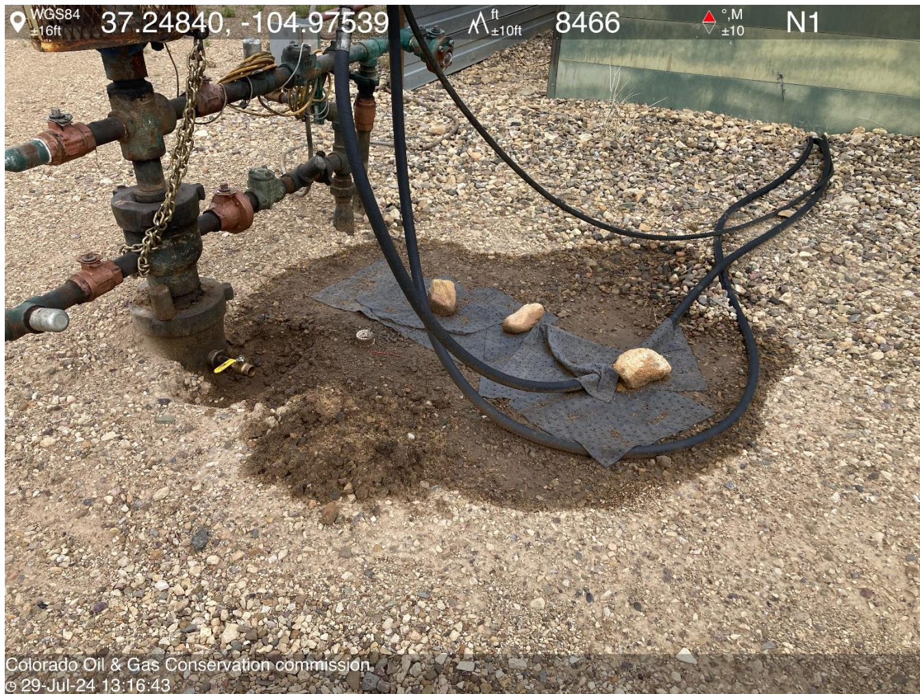
PHOTO 4: AREA OF IMPACTED SOIL NEAR WELLHEAD (APPEARS THAT LEAK HAS BEEN FIXED). REMOVE OR TREAT IMPACTED SOILS, Self-inspection, maintenance, and good housekeeping procedures and schedules PER RULE 1002..(2).D. CA DATE 8/29/2024.
