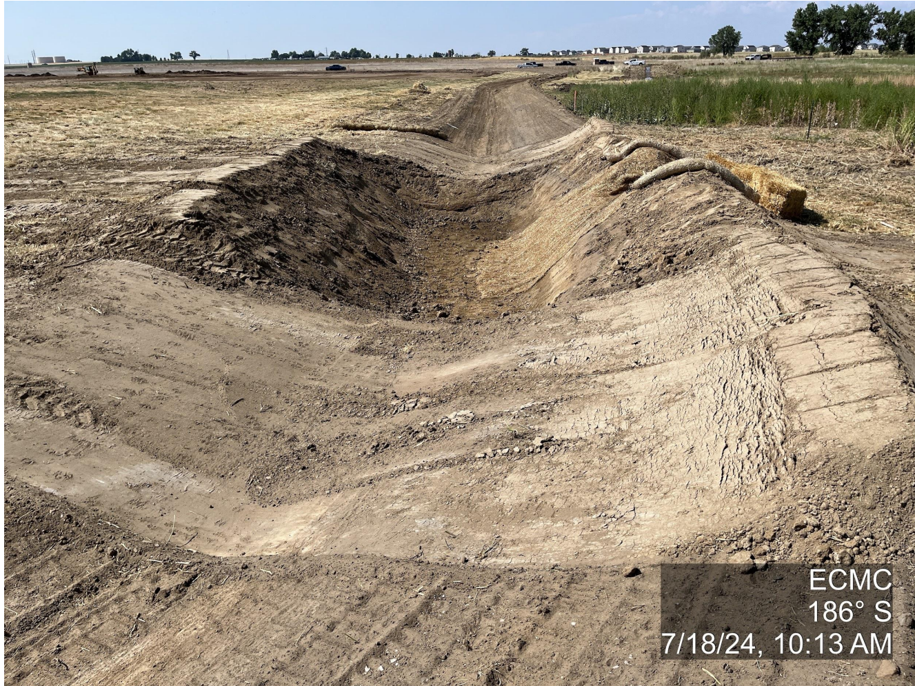
Photo 7. The photo was taken at the well location facing South. The photo illustrates a location sediment trap, with sides that appear to be appropriate and a protected outlet.
