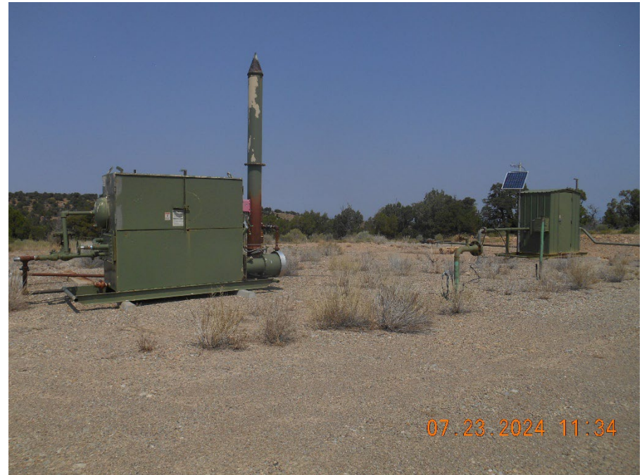
Separator and Meter housing
