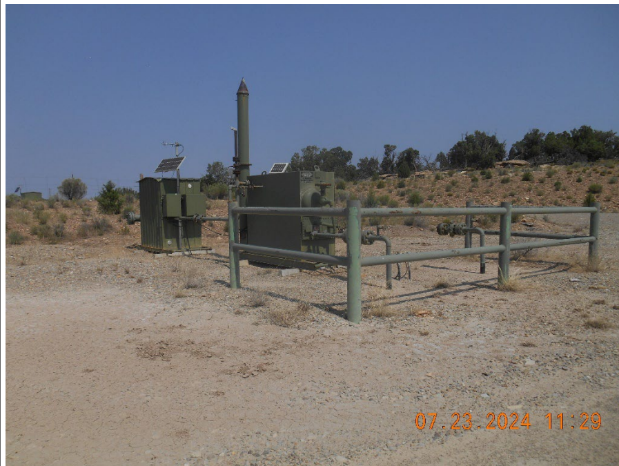
Separator and Meter housing
