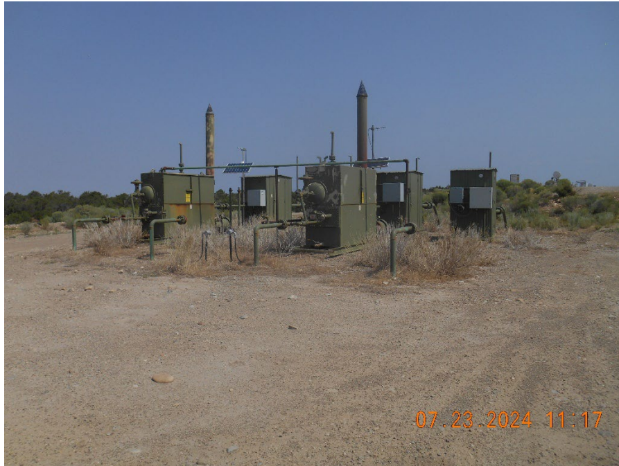
Separators & Meter housings
