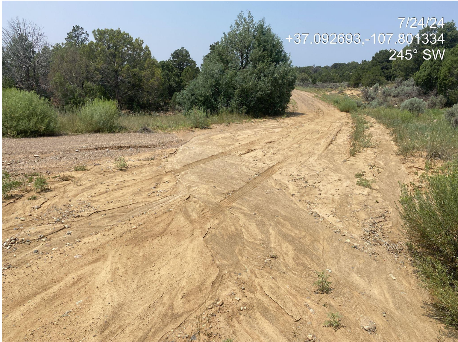
Photo 4. View of sediment deposition occurring at the well disturbance access point.
