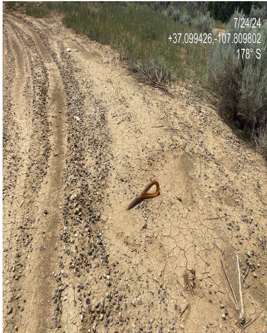
Photo 2. View of unmarked guy line anchors on location.
