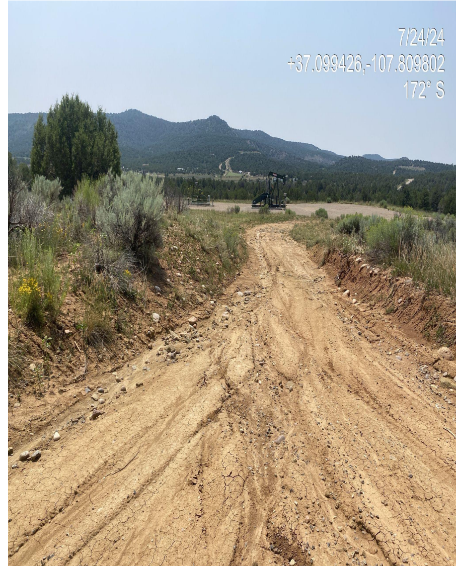
Photo 3. View of storm water and sediment transport at well disturbance and along access road.
