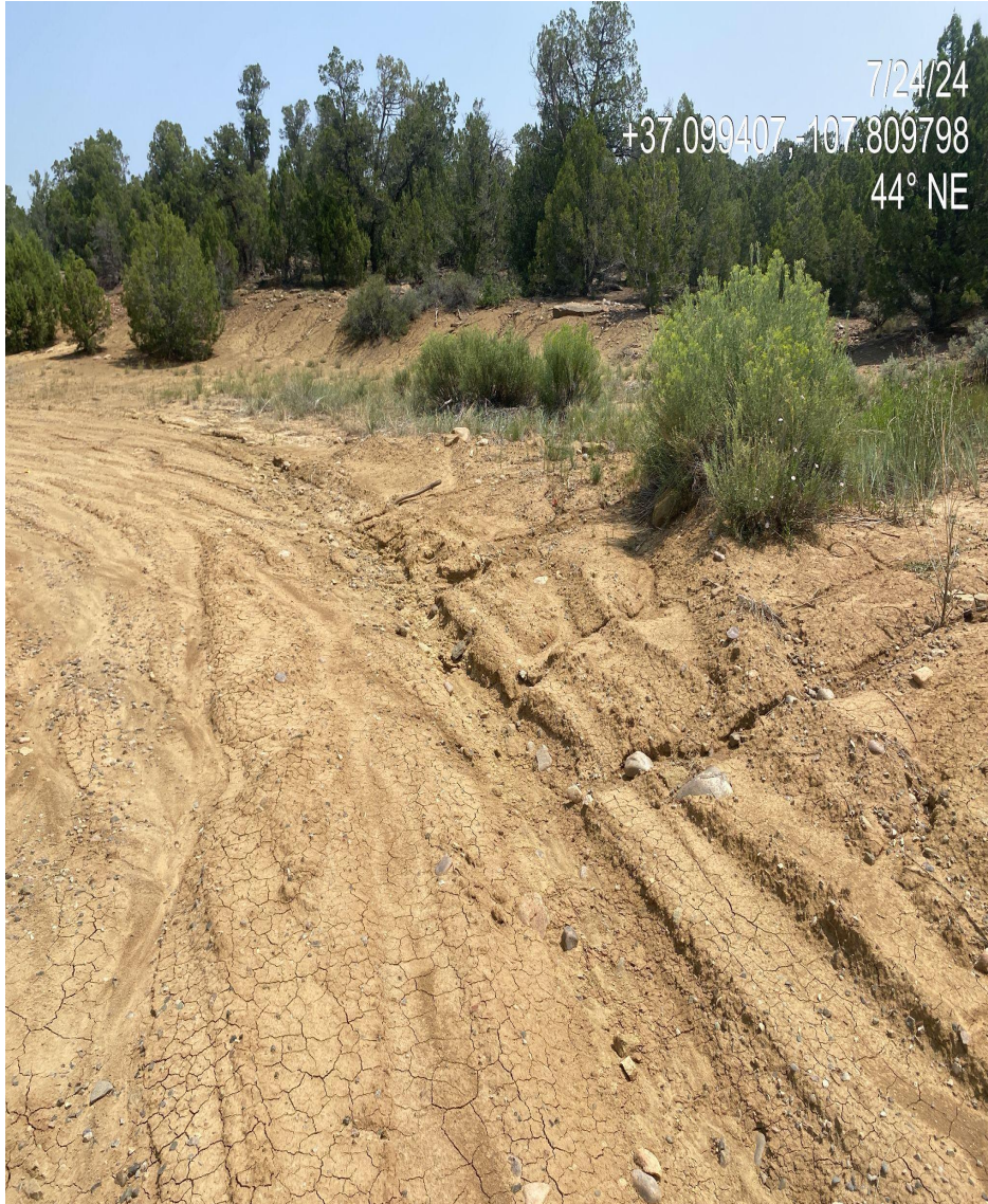
Photo 3. View of storm water and sediment transport at well disturbance and along access road.
