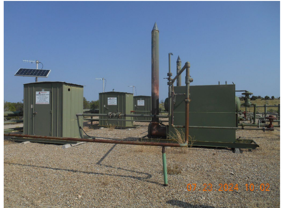
Separators & Meter housings
