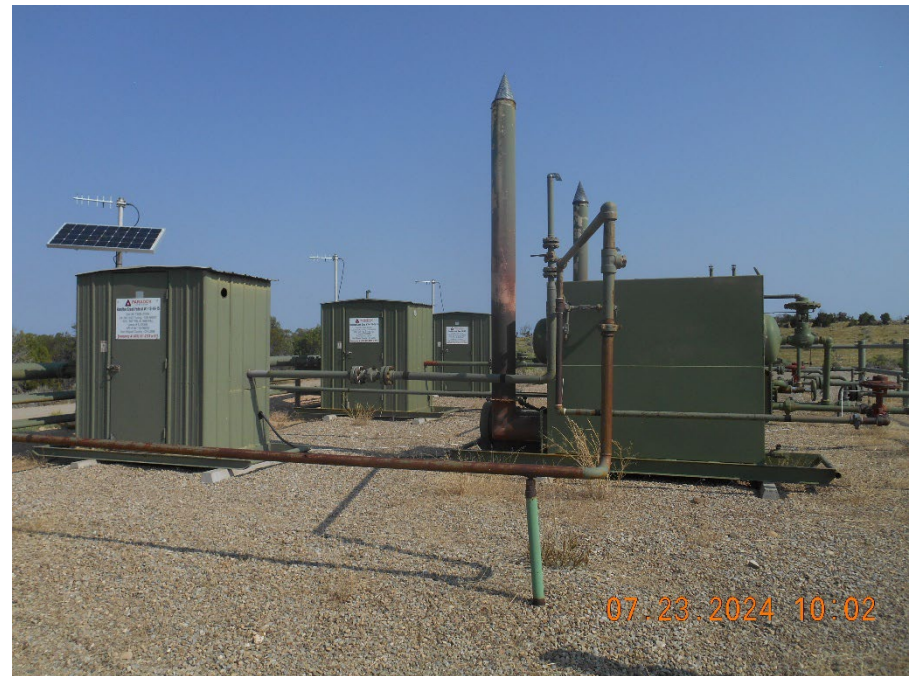
Separators & Meter housings
