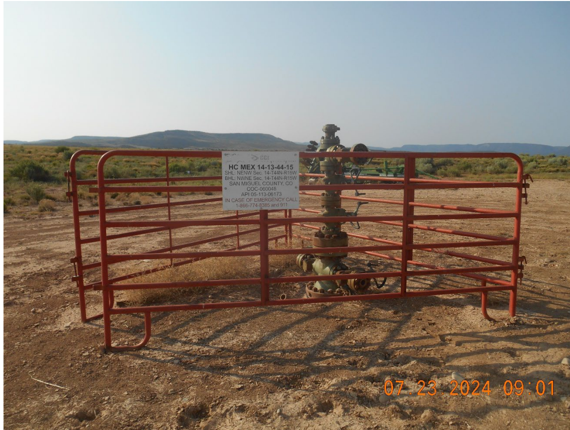
Wellhead with sign and fence. Temporarily abandoned.
