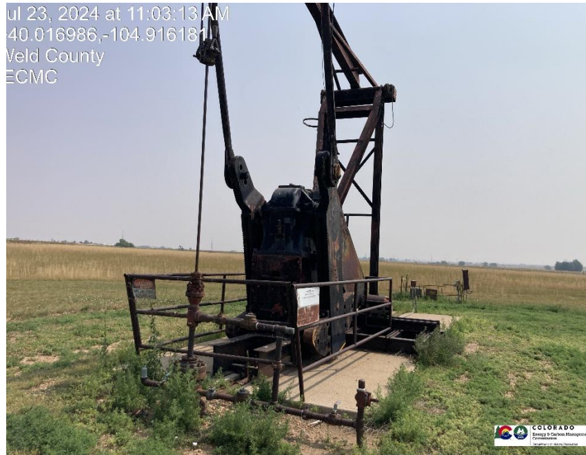
Pic 1 wellhead / pump jack
