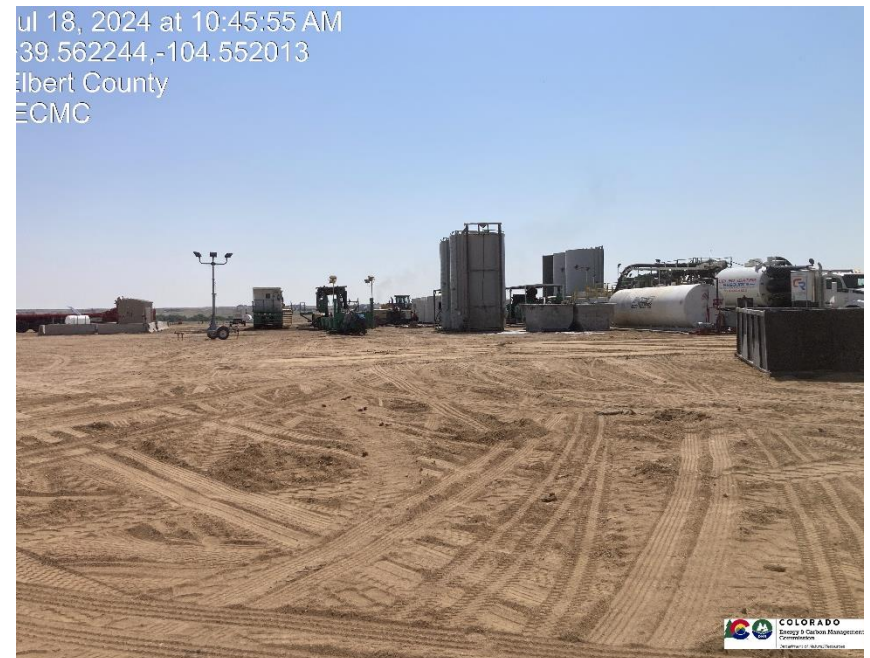
Pic 2 Cementing equipment
