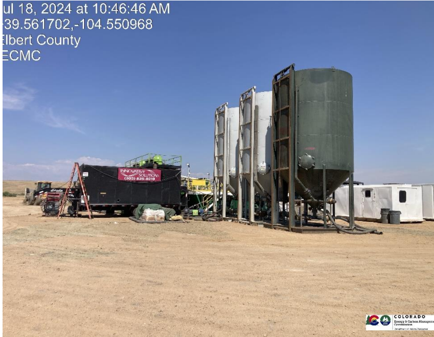
Pic 3 Chemical storage
