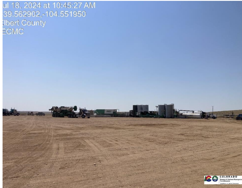
Pic 1 Cementing equipment
