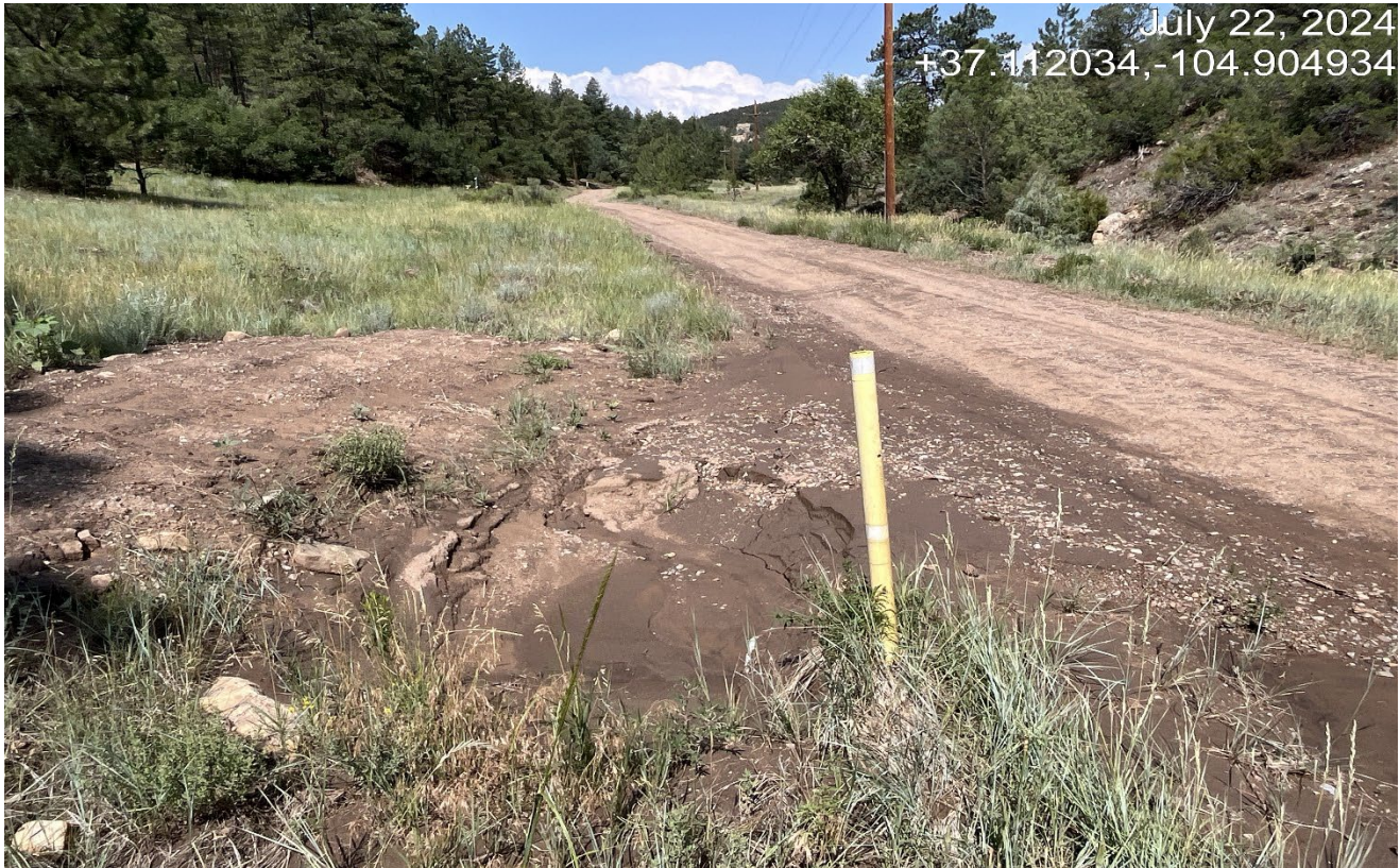
Photo 1. There is a culvert in the canyon bottom that needs to be cleaned out.
