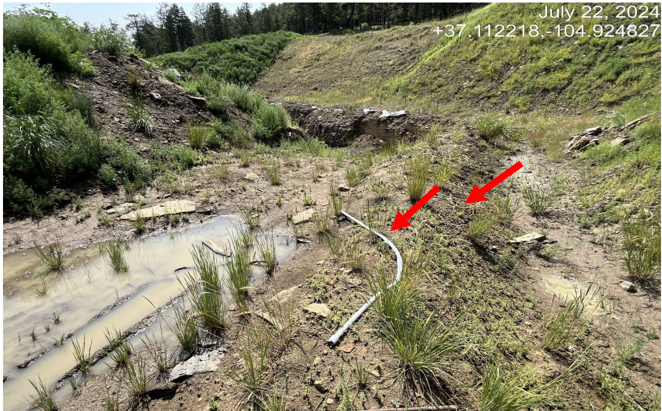
Photo 5. There is pipe and wire shown at red arrows that need to be removed..
