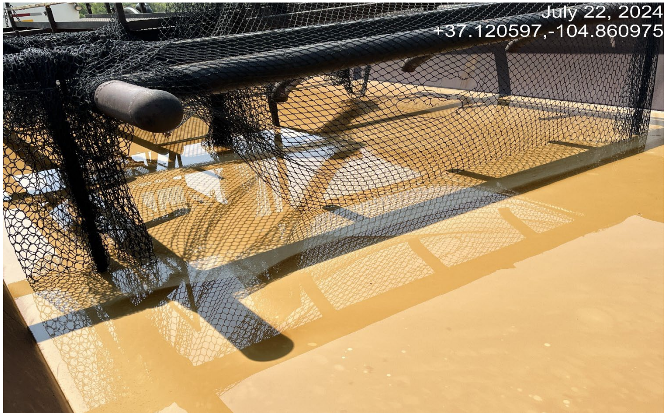
Photo 8. The netting on the open top tank is not maintained.
