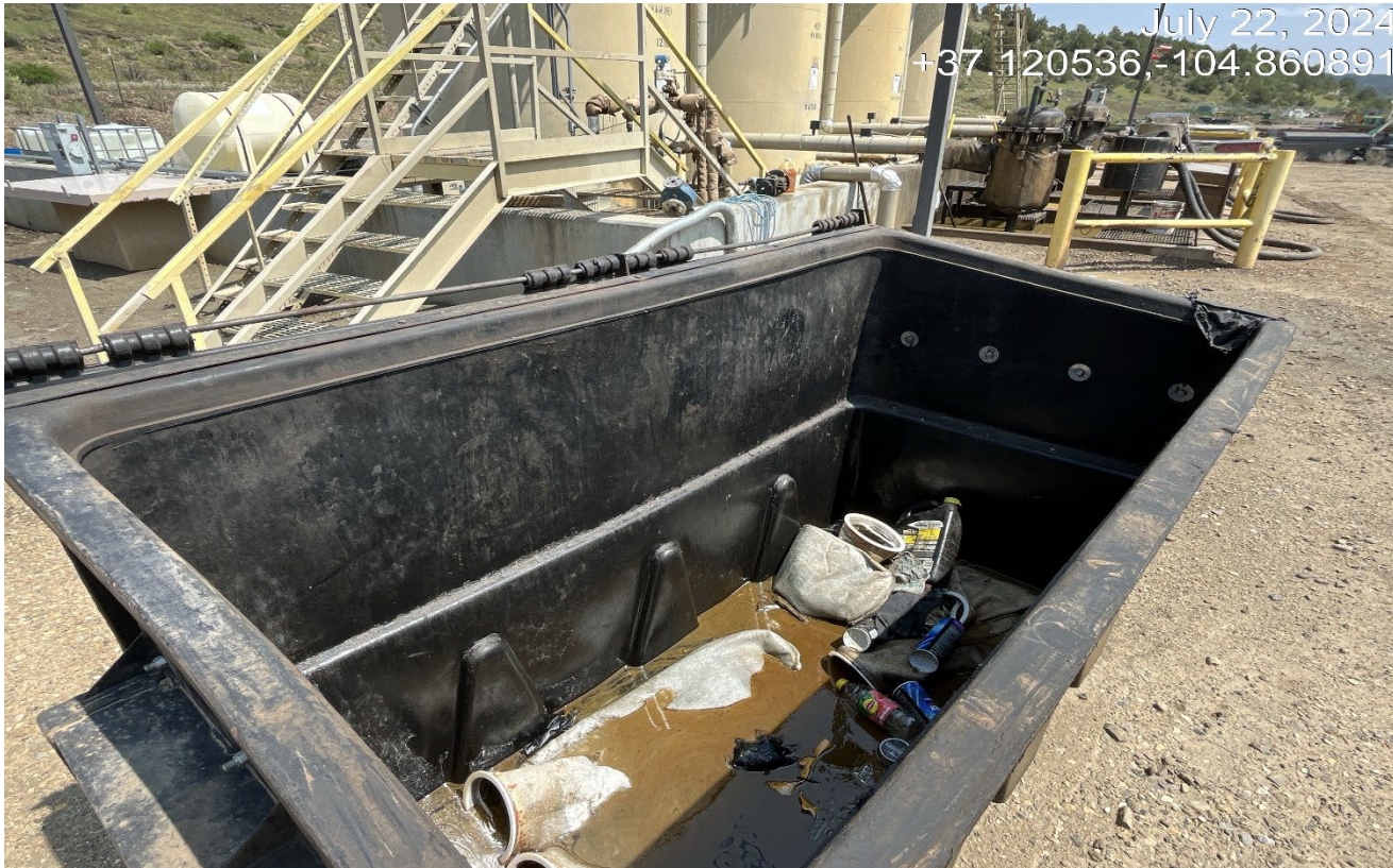
Photo 4. There is oily fluids inside this plastic container which has no netting to prevent wildlife entry.
