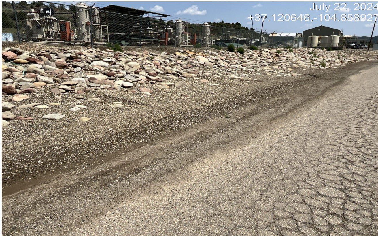
Photo 2. There is sediment that has filled in along the road side from the production facility.
