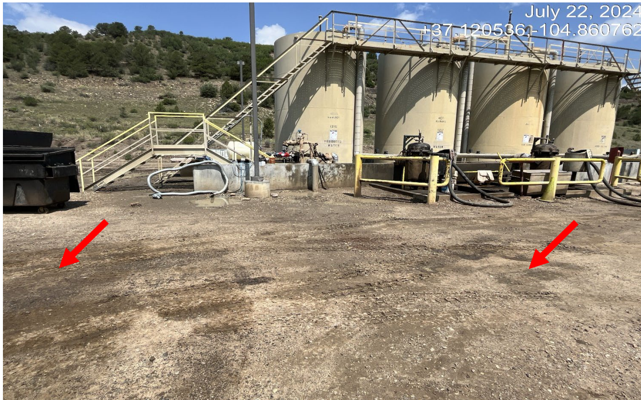
Photo 3. Facing northwest toward the tank battery. There are oil stained soils in this area that must be cleaned up.
