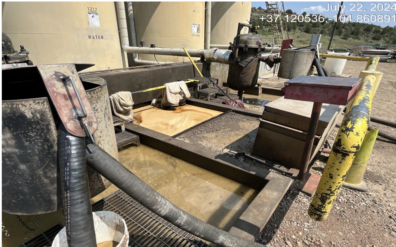
Photo 5. There is oily fluids in the secondary containment that has spilled over onto the ground. Additionally netting must be installed to prevent wildlife entry.
