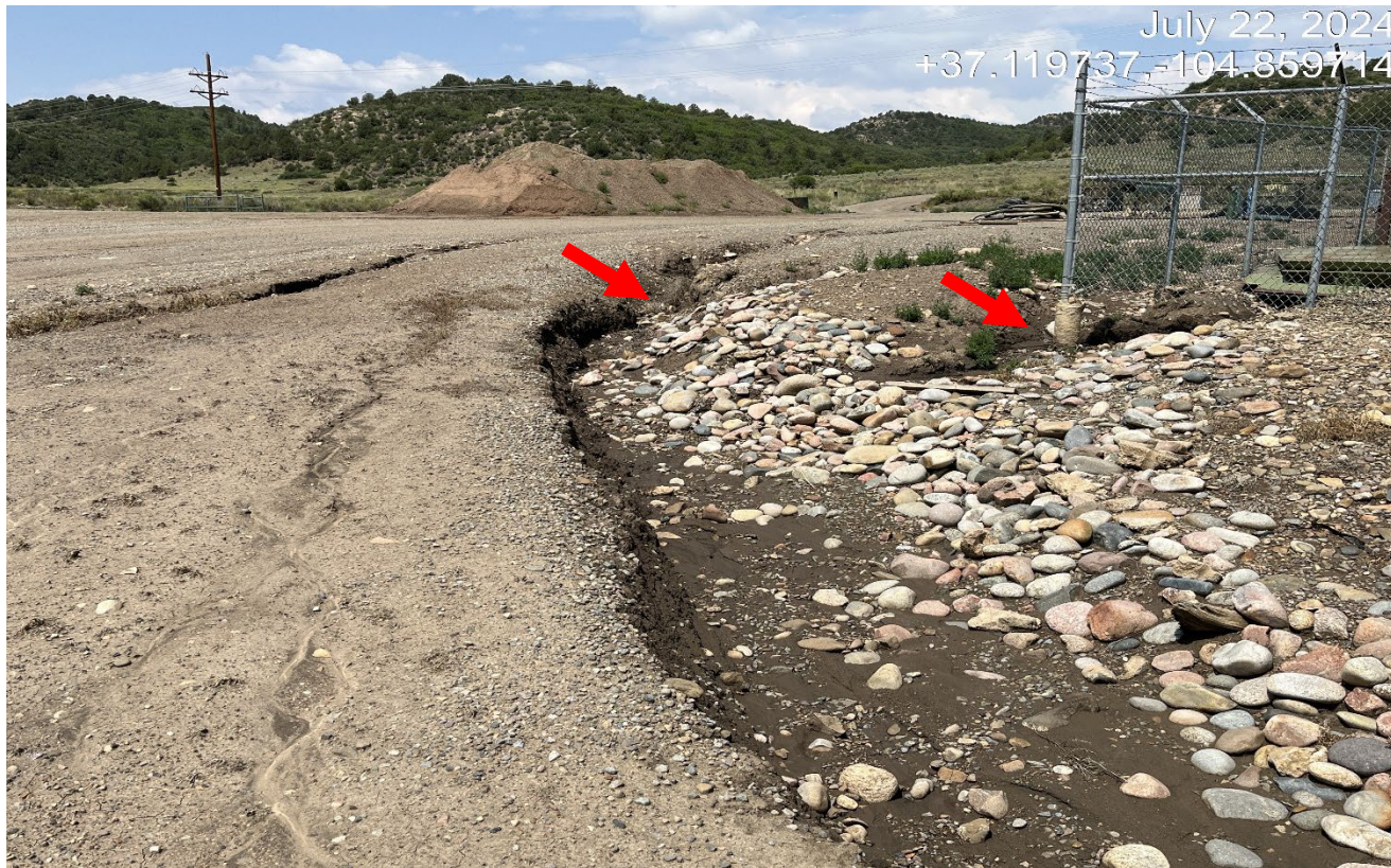
Photo 1. Facing west at the road to the production facility. There is erosion along this area and the round rock has washed out. Angular rock would be better for erosion control..
