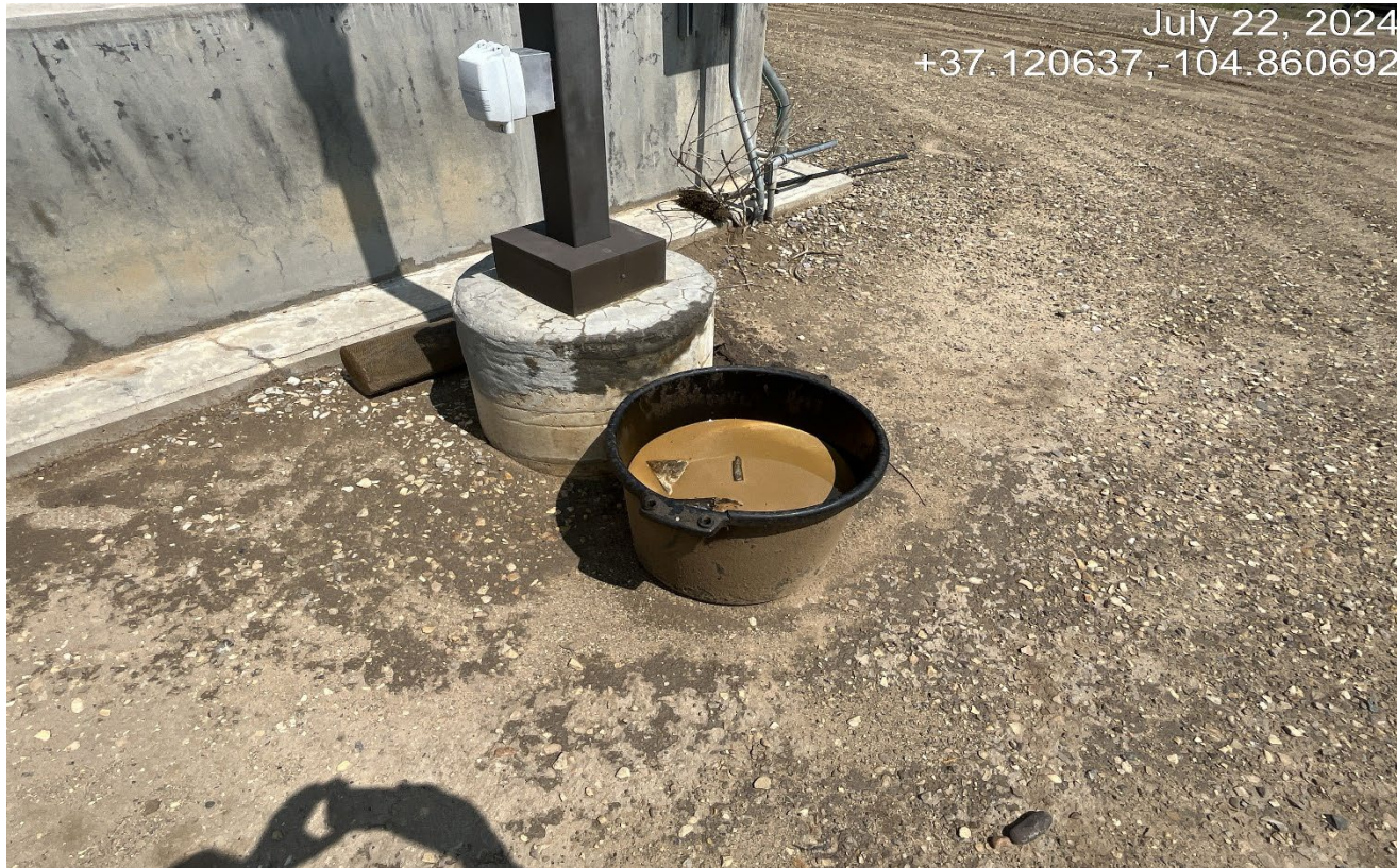
Photo 6. There is a bucket of oily fluid at the northeast side of the tank battery that needs to be disposed and contained in secondary containment with netting.
