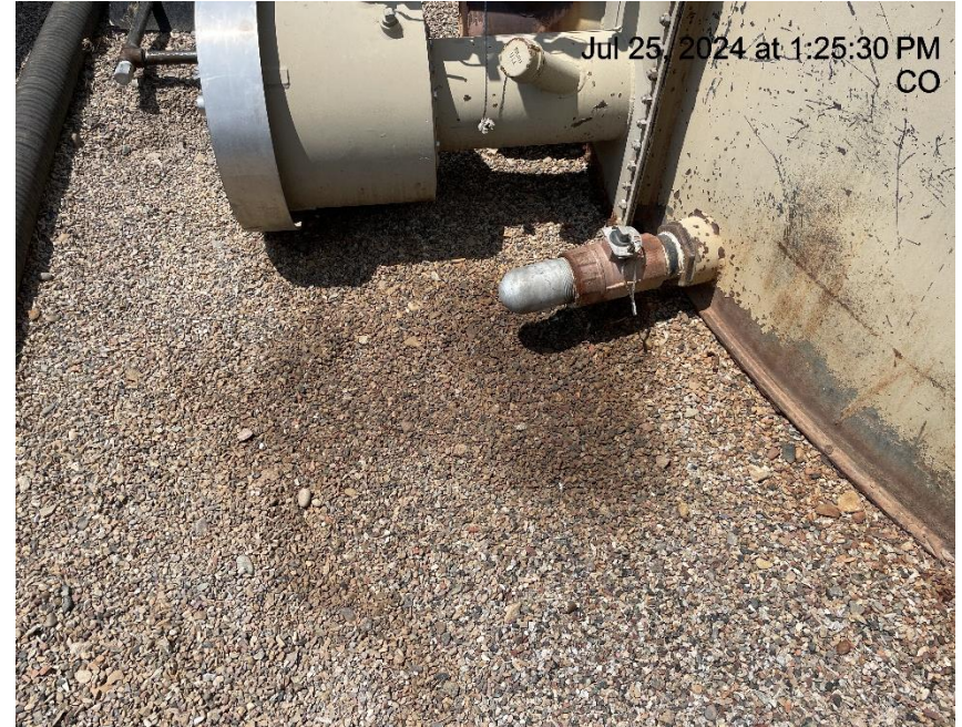
Photo # 3337 Staining in secondary containment
