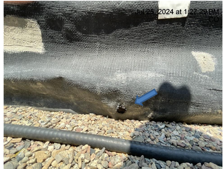
Photo # 3351 Hole in liner/liner needs maintenance
