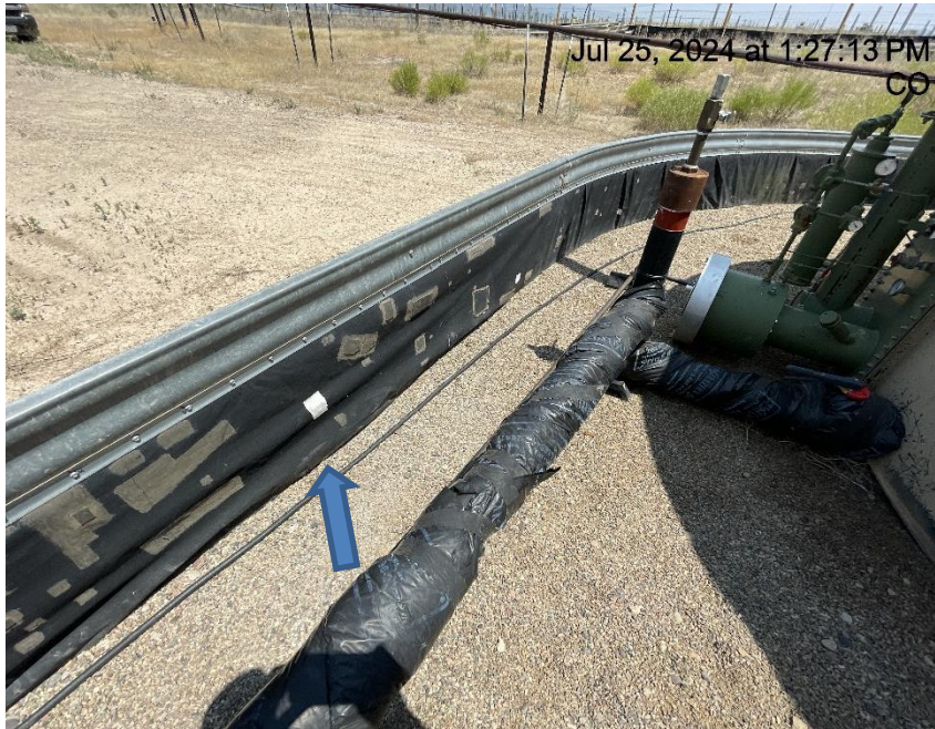
Photo # 3350 Hole in liner/liner needs maintenance
