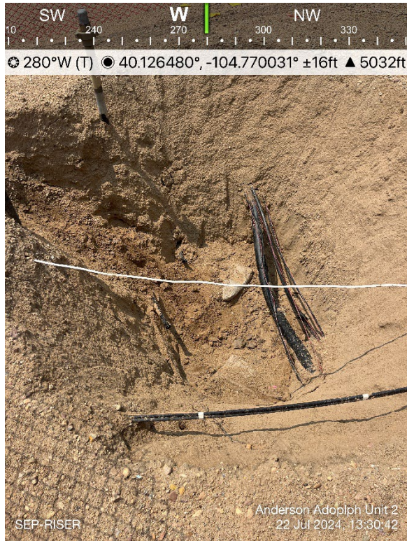
Separator Riser Excavation
