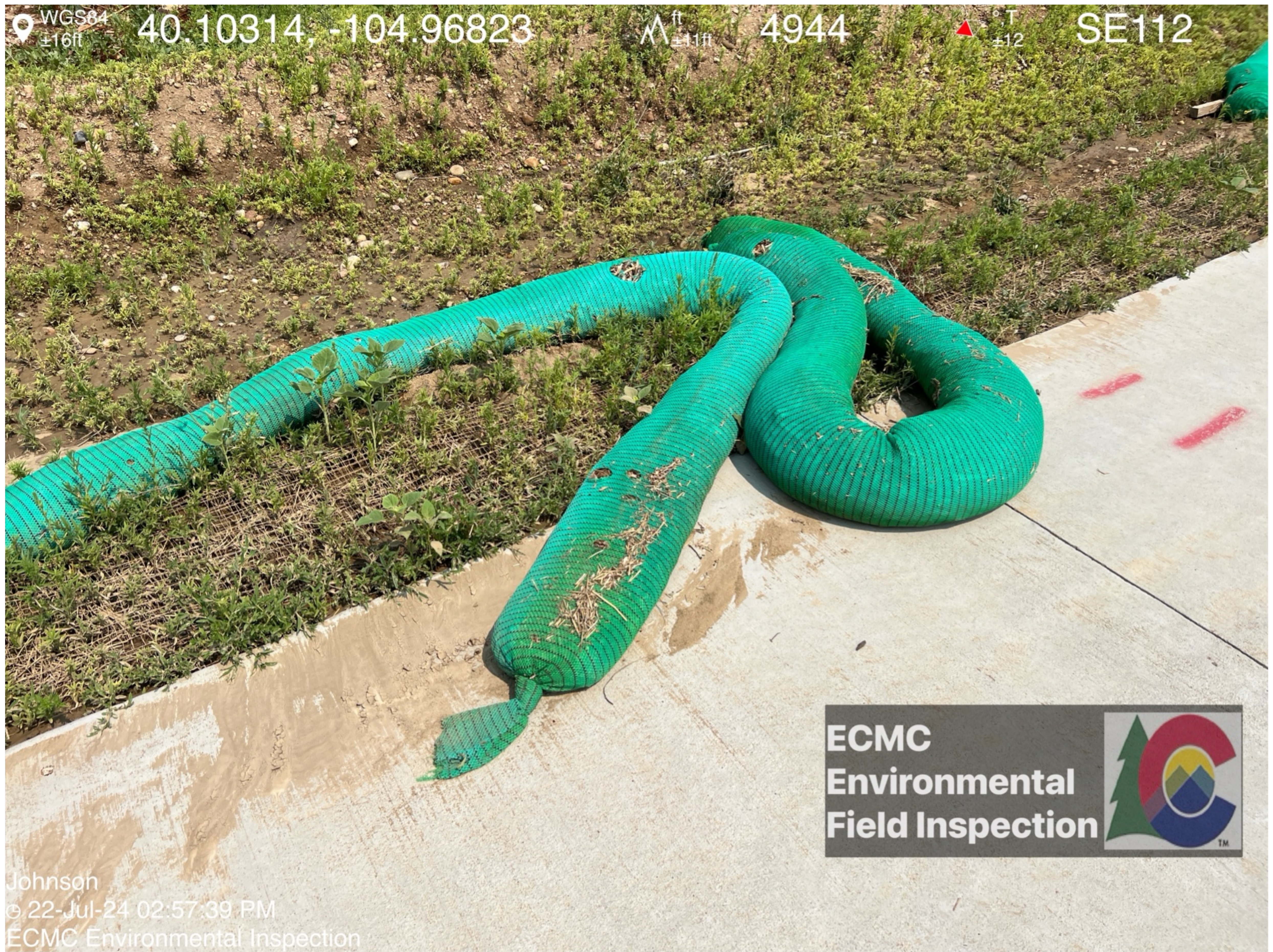
Failed/Inadequate BMPs
