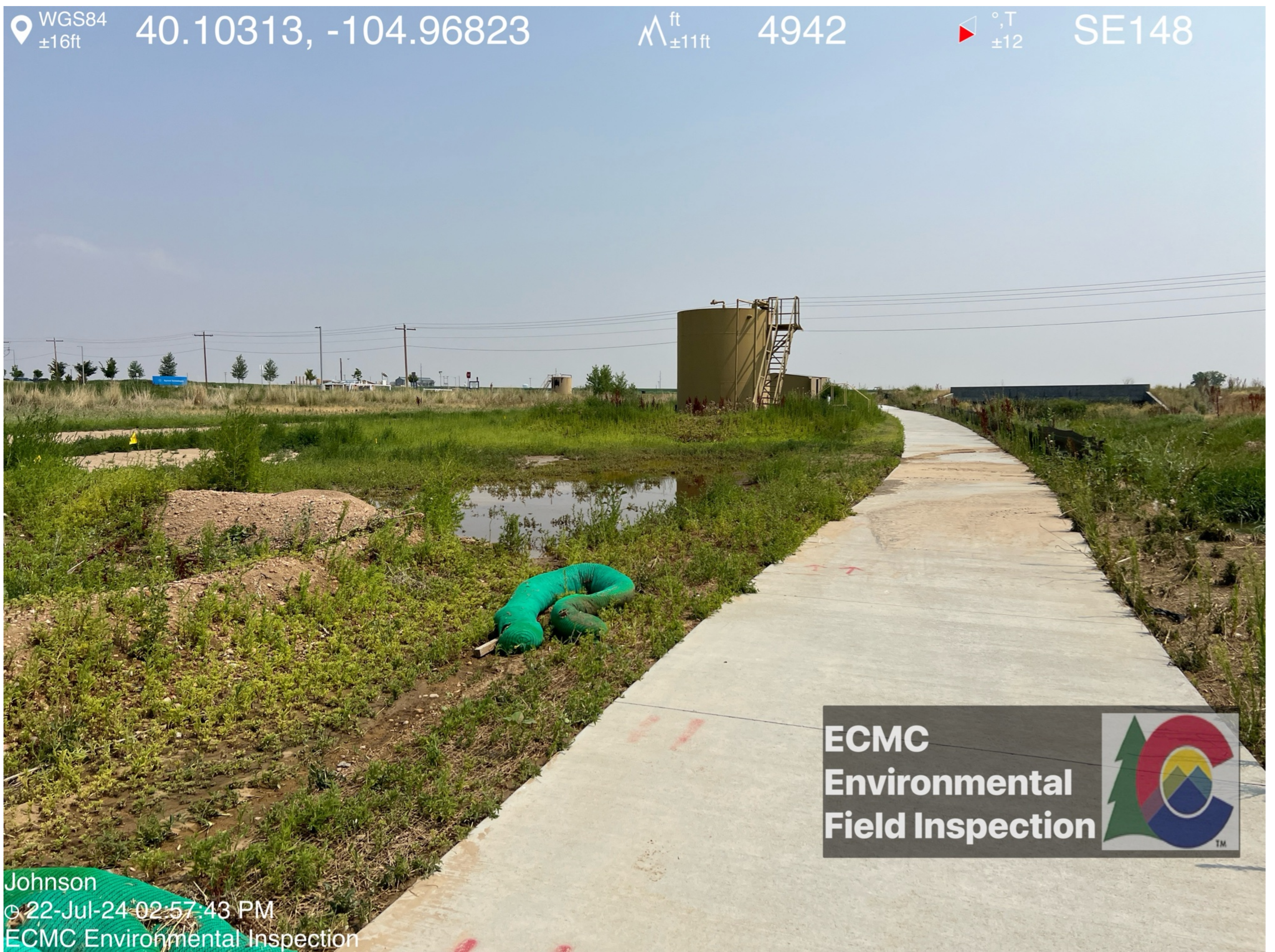
Failed/Inadequate BMPs, weeds
