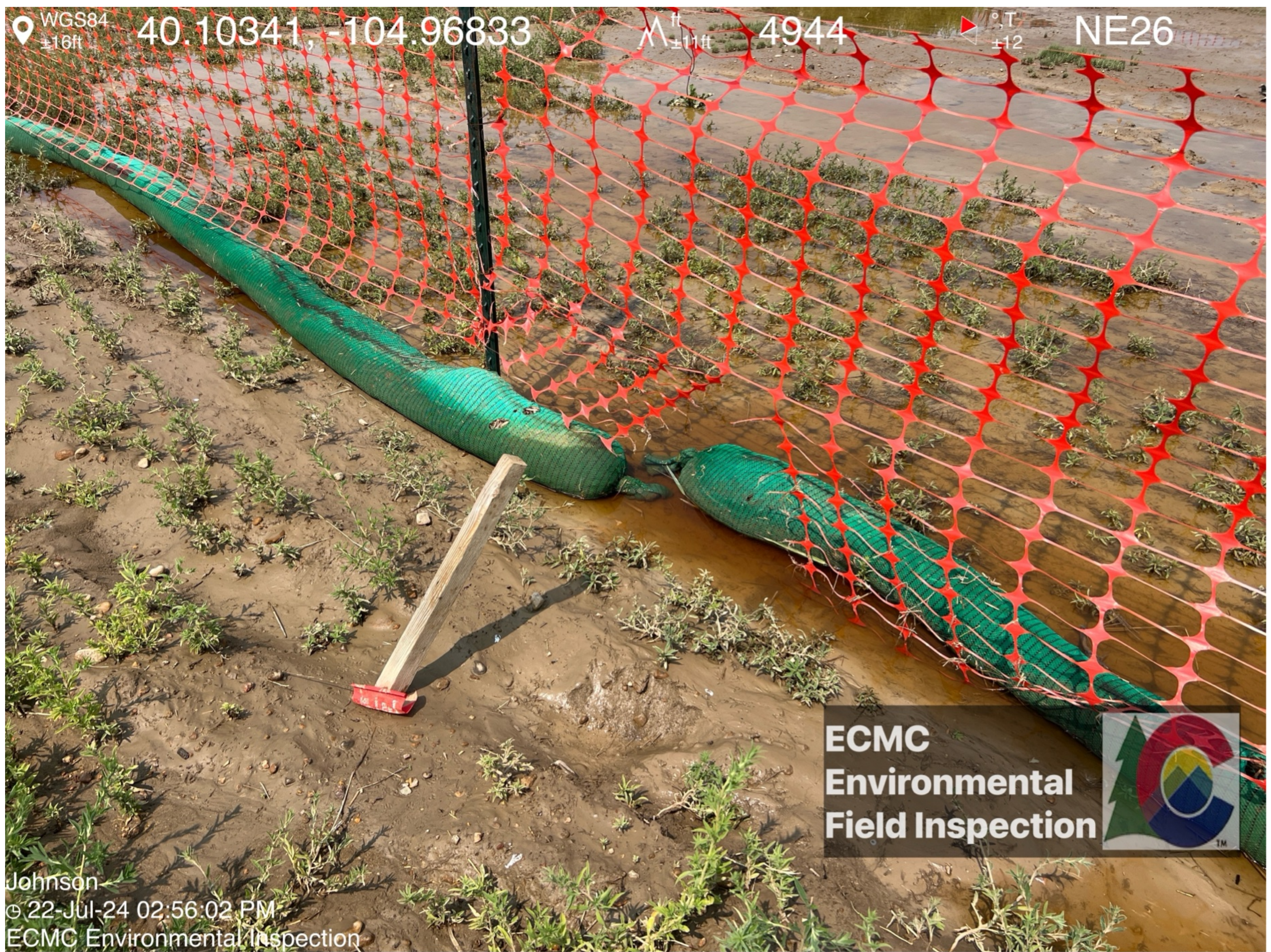
Inadequate BMPs
