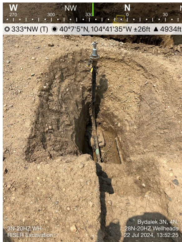
3N-20HZ Wellhead Riser Excavation
