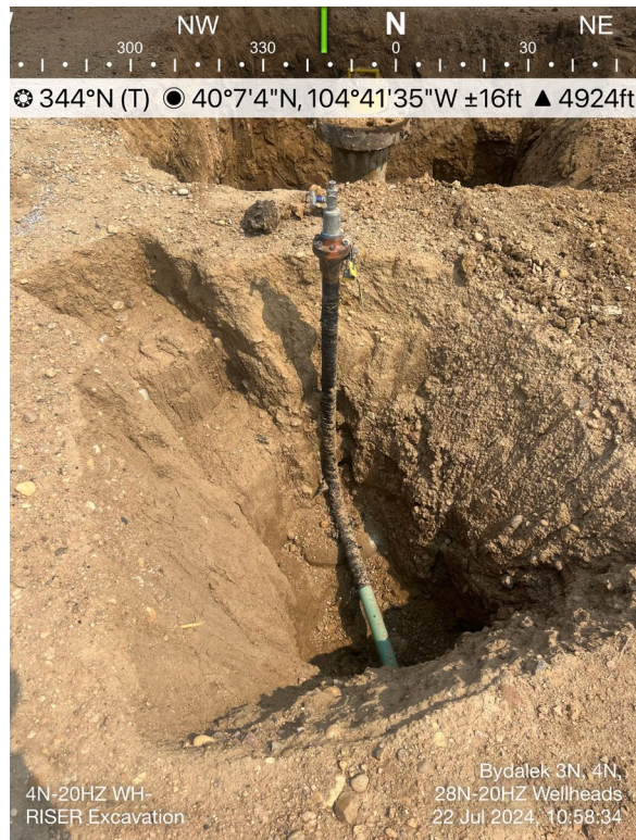
4N-20HZ Wellhead Riser Excavation
