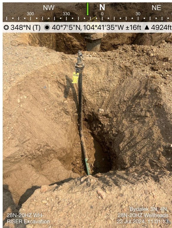
28N-20HZ Wellhead Riser Excavation
