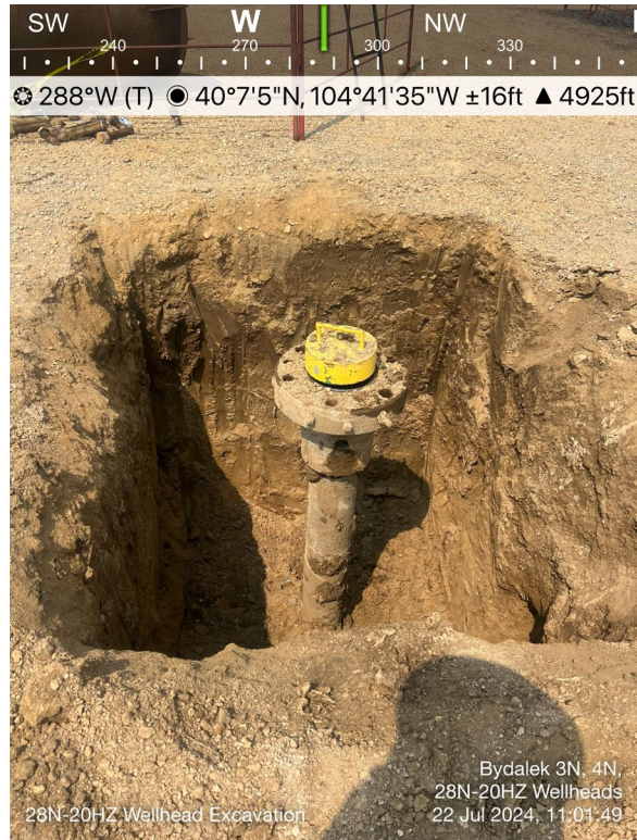
28N-20HZ Wellhead Excavation
