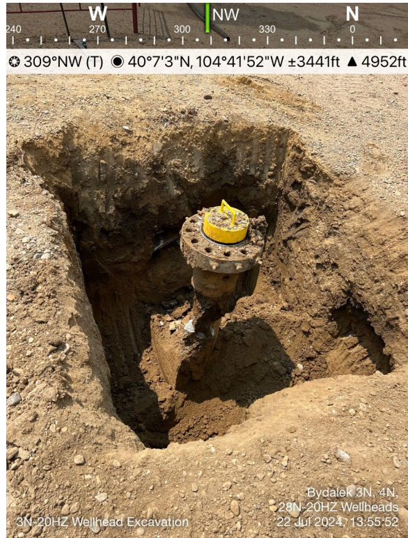
3N-20HZ Wellhead Excavation
