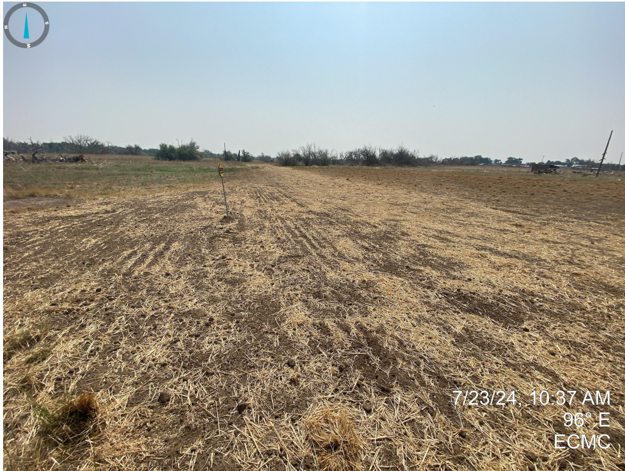
Photo 2. Taken from the western portion of the former tank battery location. It appears that the Operator has performed additional reclamation work with evidence of drill rows and straw crimped mulch. This location will be inspected at a later date to verify compliance with Rule 1004.
